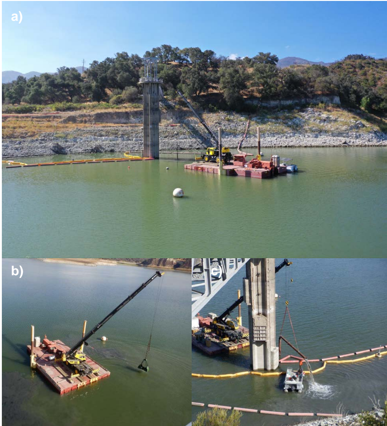
Figure 2: a) work barge dredging around the intake tower (J.Waller); b) clamshell bucket utilized for dredging around the berm and around the intake tower; c) airlift utilized for finer scale dredging around the intake box.
