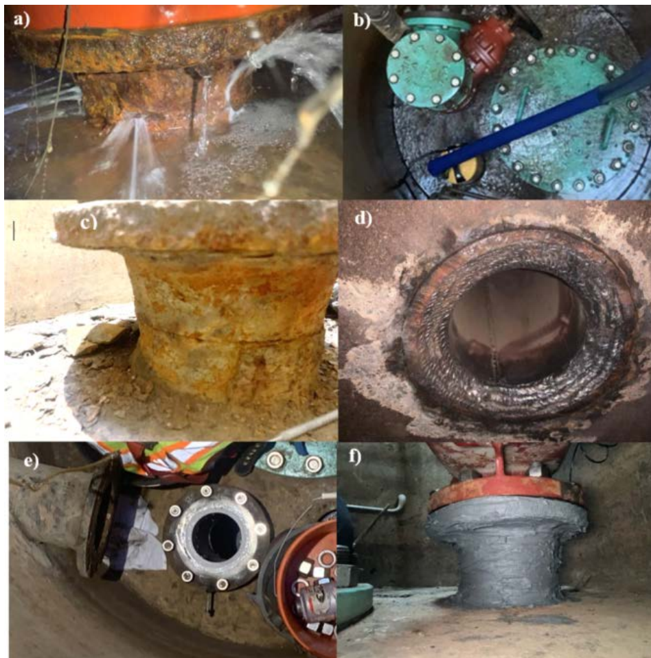
Figure 3. 639+50 – Blowoff Riser Repair – a) leak observed on 10/20; b) leak pumped out on 10/20; c) circumferential crack in the steel pipe around at weld; d) bottom weld of the 5-inch diameter steel sleeve into the 6-inch diameter pipe; e) all bare metal surfaces coated after welding; f) outside of the pipe was cleaned to bare metal and coated with a super metal epoxy.
