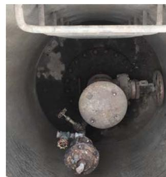
*Corroded air-vac at Station 676+67*
