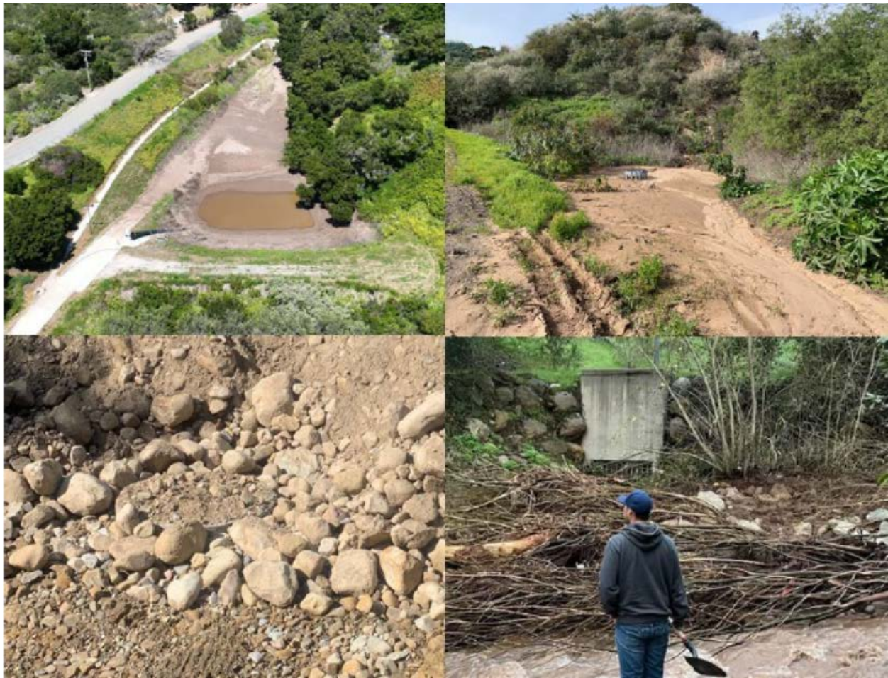
Figure 1. (a) Lauro Main Debris Basin, (b) San Roque Road Debris Basin above Lauro Reservoir, (c) Toro Canyon Blowoff, (d) Carpinteria Toe Drain
