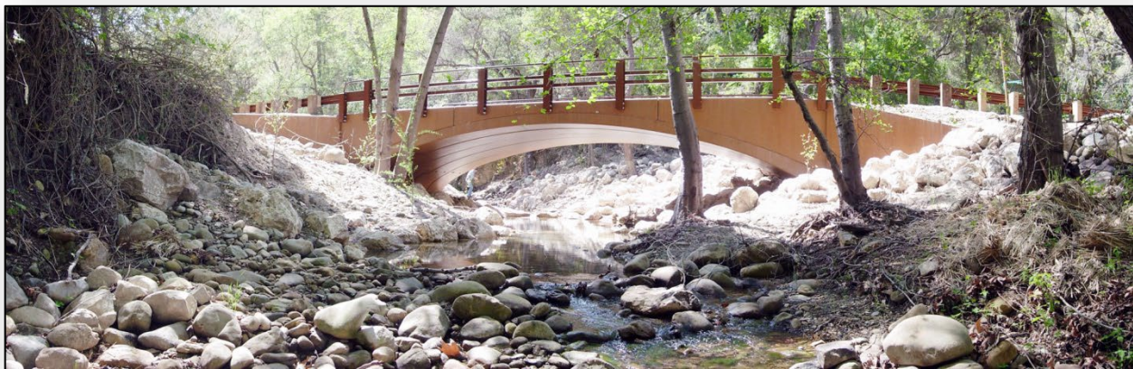
Quiota Creek Fish Passage Project
