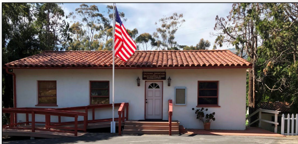
Cachuma Operation and Maintenance Board Meeting Room
