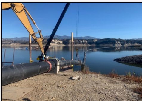
Secured Pipeline Project Staging Area
