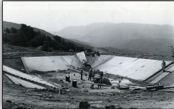
Construction of Bradbury Dam
