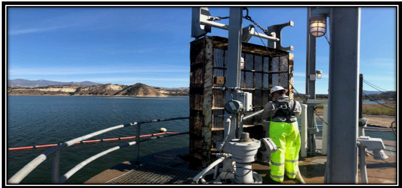
North Portal Intake Tower
