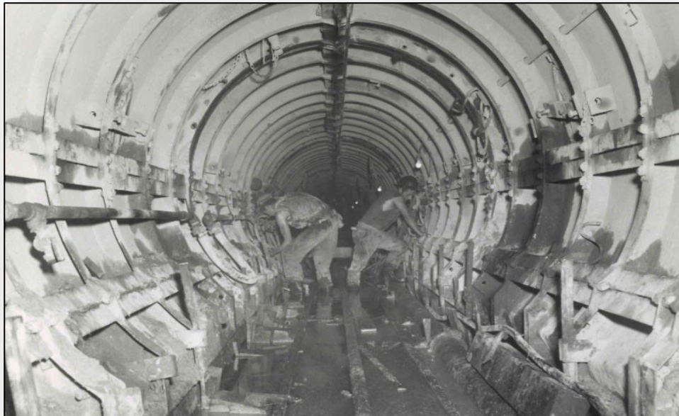
Tecolote Tunnel Construction
