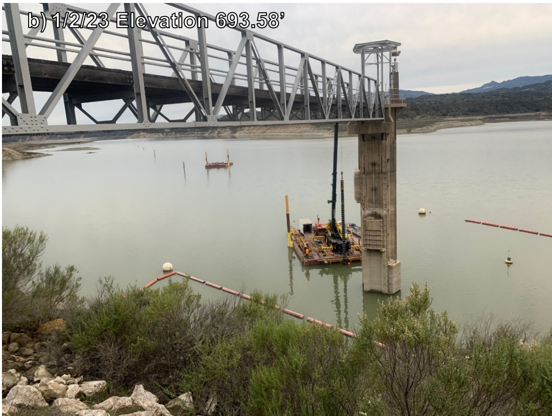
Figure 9: a) contractor setting up to drive piles at the intake tower on the 1/2/23 holiday with the lake at 693.58'; b) intake tower on 1/10/23 following 12.5" of rain at Cachuma Lake which resulted a 32.25' rise in a 24-hour period which exceeded the previous historical single day change by 10 feet.
