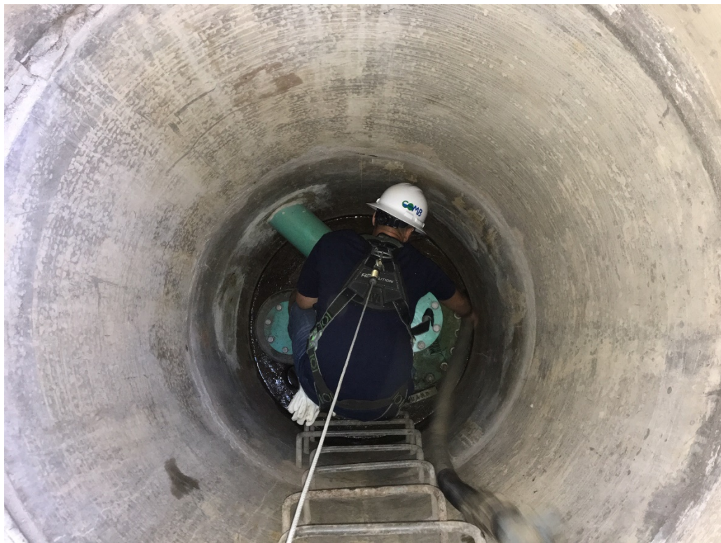
Structure maintenance and valve exercising at Blowoff 27+80
