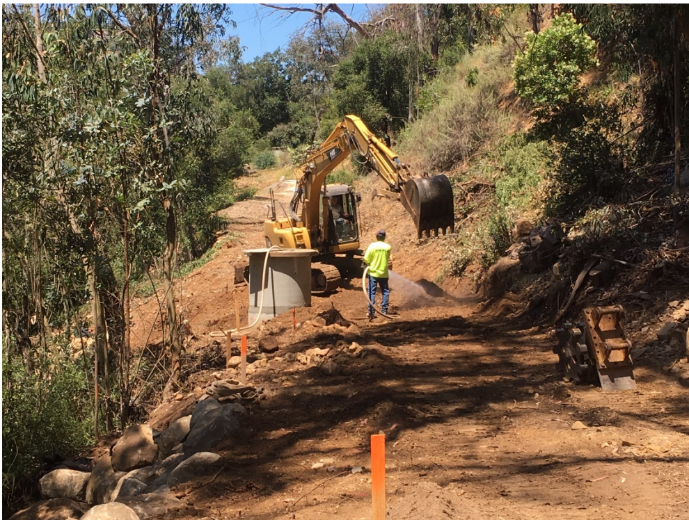
Potholed top of grout band at joint to confirm South Coast Conduit location. Pipe joint in good condition.
