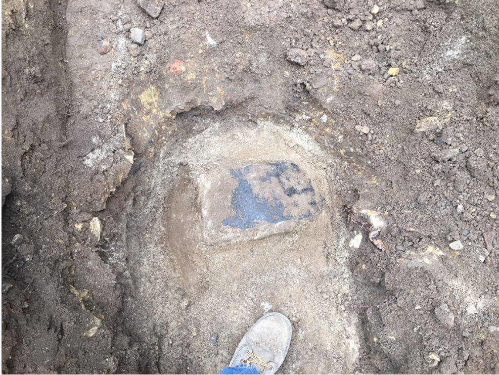
Potholed top of grout band at joint to confirm South Coast Conduit location. Pipe joint in good condition.
