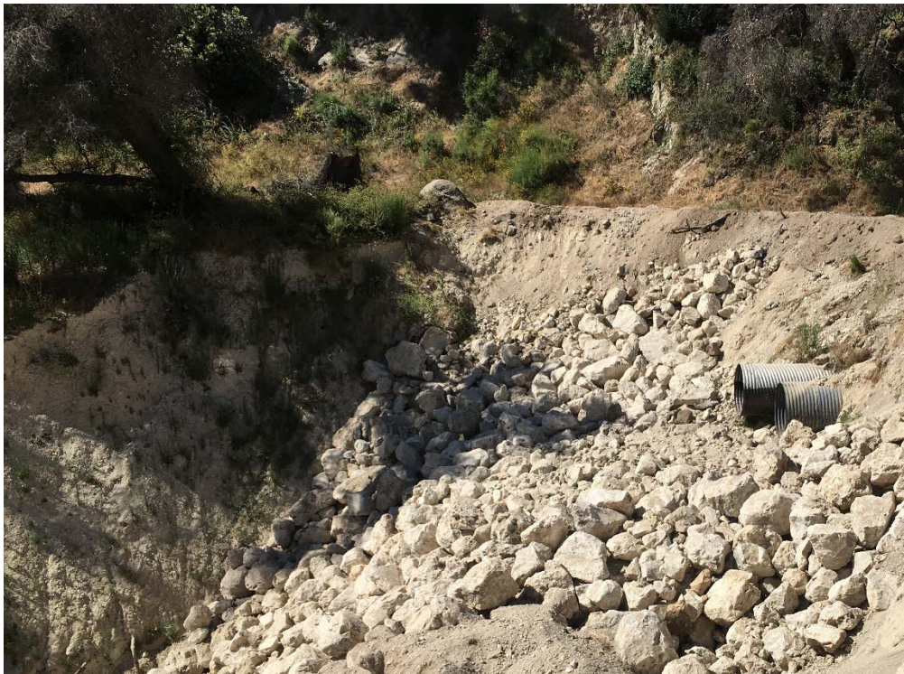
Rock slope protection installed below culverts on North Portal Access Road
