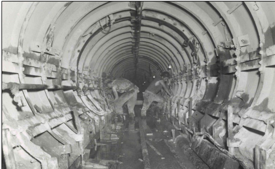
Tecolote Tunnel Construction
