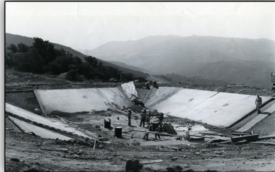
Construction of Bradbury Dam
