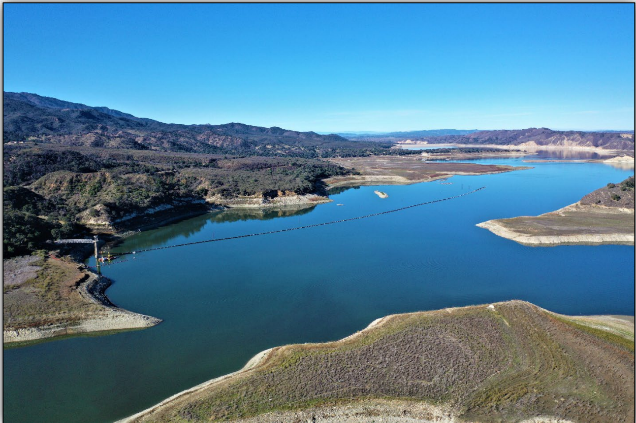
Lake Cachuma Tecolote Tunnel Intake Tower Secured Pipeline Installation (December 2022)
