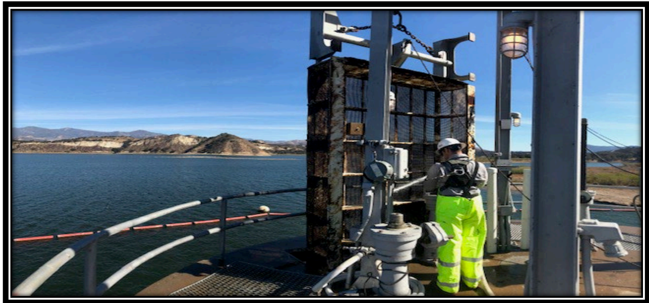
North Portal Intake Tower
