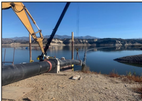
Secured Pipeline Project Staging Area
