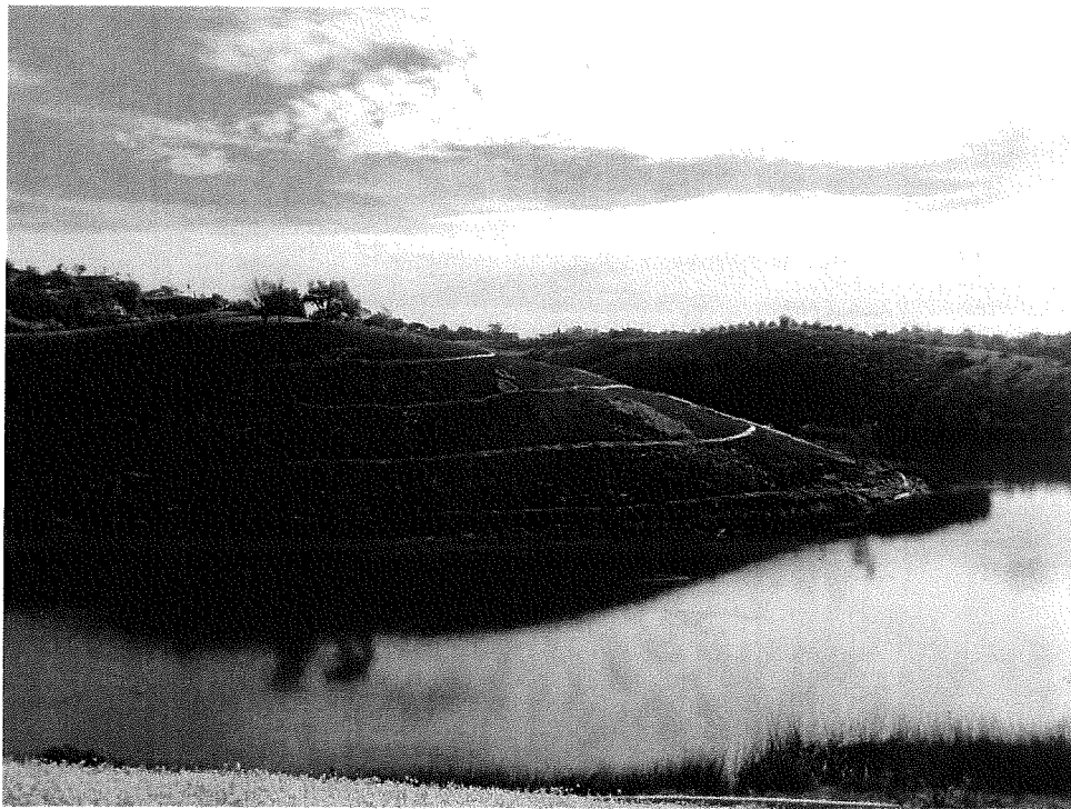
Picture 4 – Erosion control installation 100% complete, December 15th 2009
