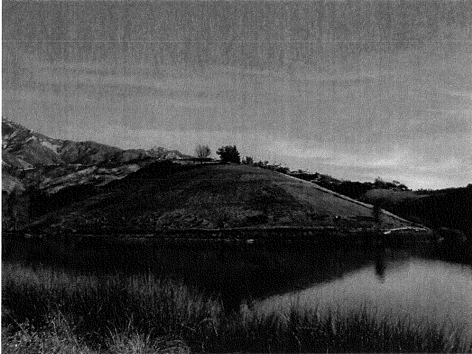
Picture 5 – Hydromulching and seeding 100% complete, December 18th 2009
