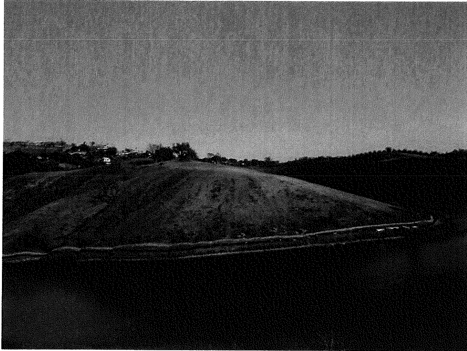
Picture 3 – Logging along eastern slope 100% complete, November 18 th 2009
