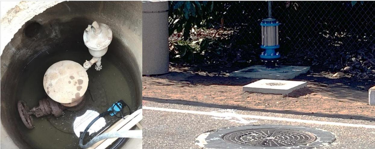
**Figure 3.** AVAR Structure 874+00 – Left – original subgrade AVAR valve with unknown function in Highway 192. Right - AVAR valve replaced and raised above grade.
