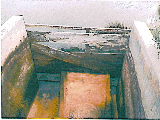
Stop Logs (Before)
