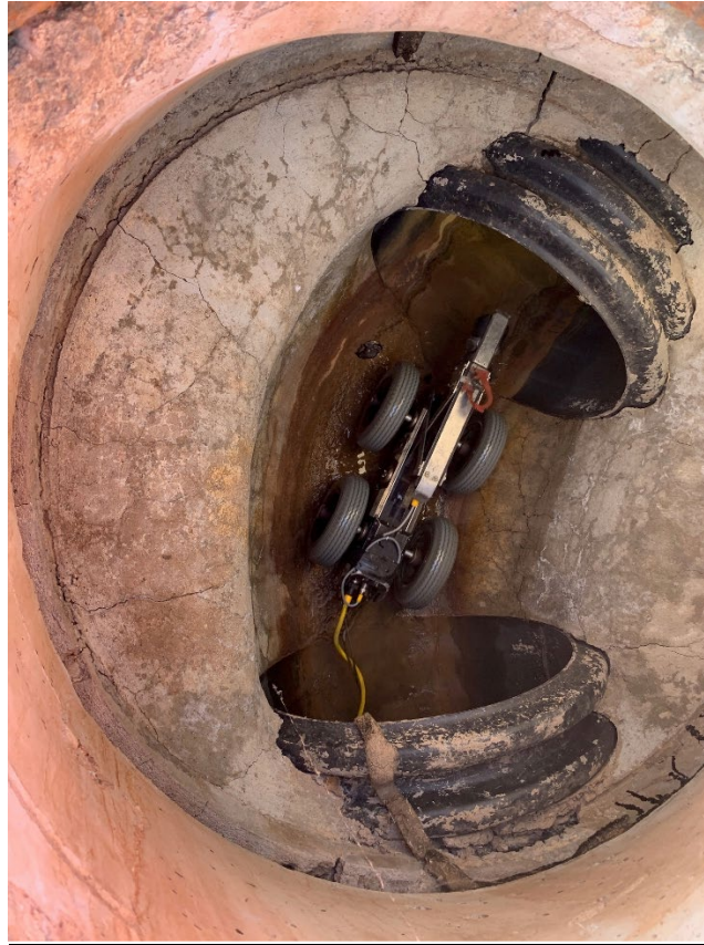
Performance Pipe Technologies camera rover inspection around Lauro Reservoir
