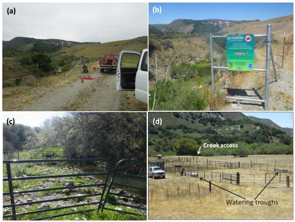
**Figure 80:** Salsipuedes Creek Cattle Exclusionary Fencing Project; (a) installation of the fencing, (b) signage on the fencing after installation, (c) cattle watering corridor showing cattle impacts to the stream within and not outside of the corridor, and (d) off-channel watering troughs.
