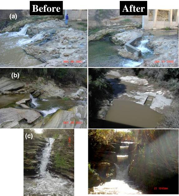
**Figure 53:** Fish passage and habitat restoration at (a) Hwy 1 Bridge on Salsipuedes Creek (completed in 2002), (b) Jalama Road Bridge on Salsipuedes Creek (completed in 2004), and (c) Cascade Chute barrier on Hilton Creek (completed in 2005).
