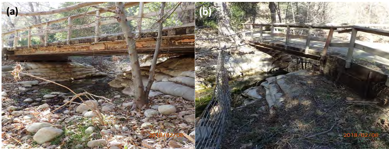
Figure 3: View of Quiota Creek Crossing 8 project location showing (a) the upstream view of the dilapidated bridge and (b) the downstream view of the dilapidated bridge.
