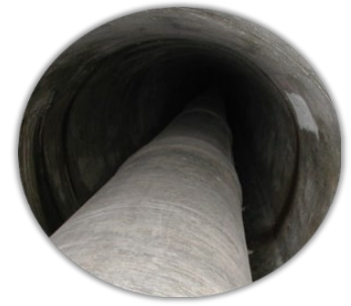
Figure - Sheffield Tunnel and Pipeline
