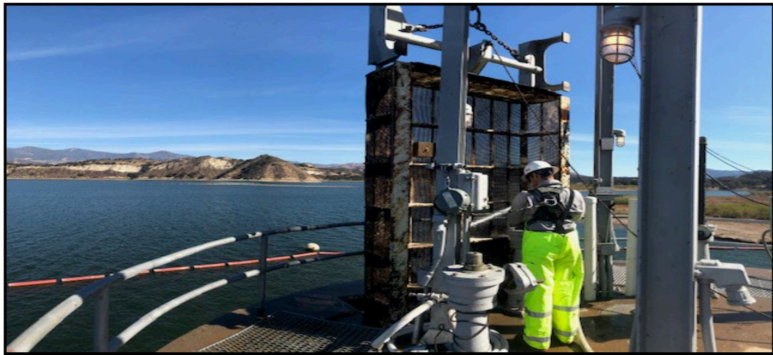
North Portal Intake Tower
