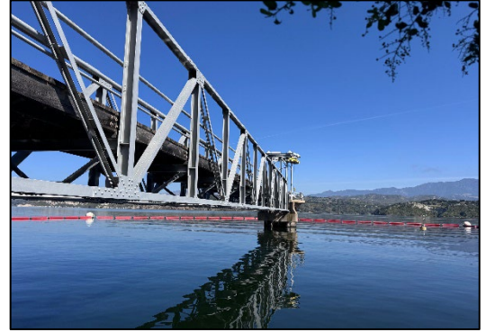
North Portal Intake Tower (April 2026)
