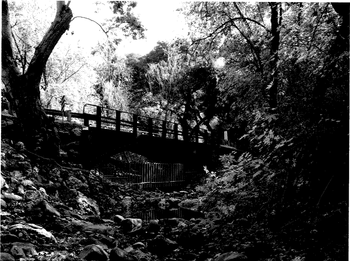
Figure 2: Quiota Creek Crossing 7, completed project condition looking upstream towards the bridge and cattle exclusion fencing
