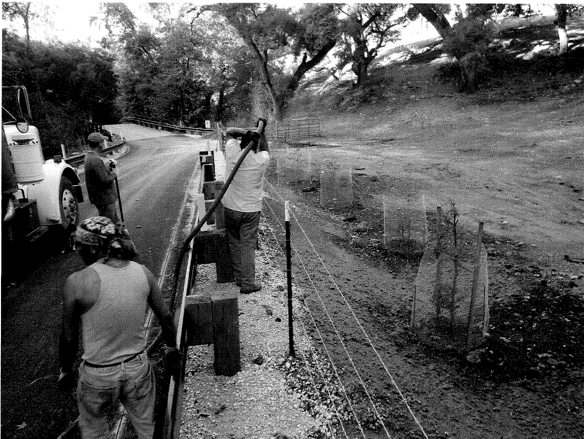
Figure 4: Hydro mulching and seeding (11/20/12).
