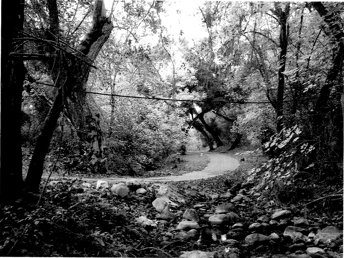
Figure 1: Quiota Creek Crossing 7, pre-project condition.
