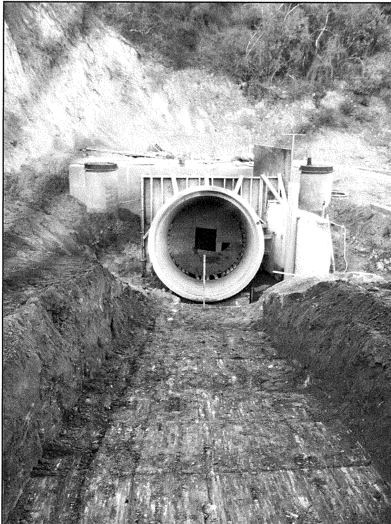
Constructing Tunnel Access
