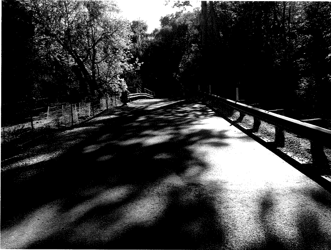
Figure 7: Looking south across the bridge (11/19/12).
