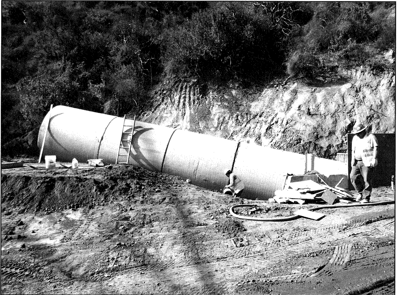
Constructing Tunnel Access
