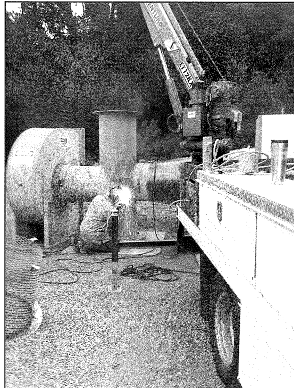
Installing Blower at North Portal
