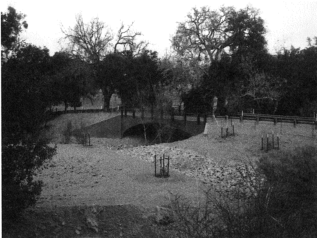
Figure 2: Completed project on 1/3/14.
