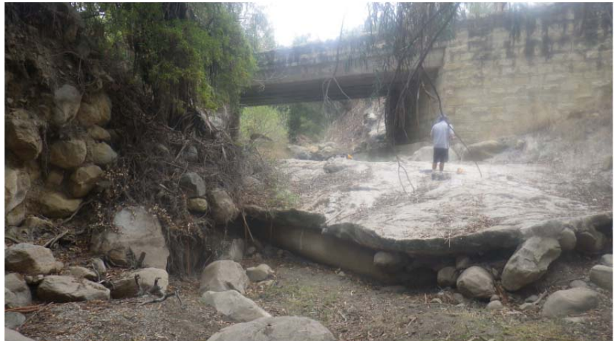
Figure 6: Mission Creek at Highway 192 showing the fish passage impediment, SCC and protective concrete on top.
