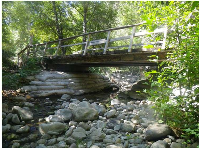
Figure 2: Quiota Creek on Refugio Road showing upstream view of Crossing 8.
