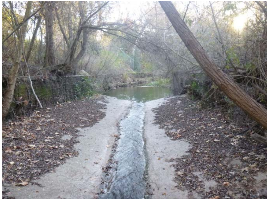
Figure 7: Maria Ygnacio Creek at San Marcos Road showing the fish passage impediment where the SCC crosses the creek with protective concrete on top.
