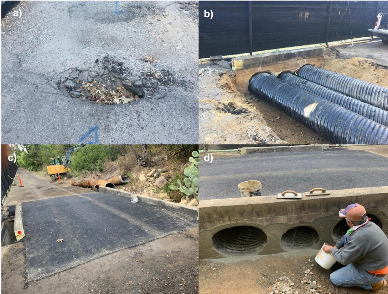
**Figure 4.** Sheffield Control Station Access Road Culvert Repair - a) Sinkhole starting to form in roadway over the South Coast Conduit alignment due to collapse culvert; b) new polymer-coated corrugated steel culverts that should better resist future corrosion; c) slurried and paved portion of the access road over the new culverts. *Note: the rusted condition of the corroded culverts in the background;* and d) repair of headwall.
