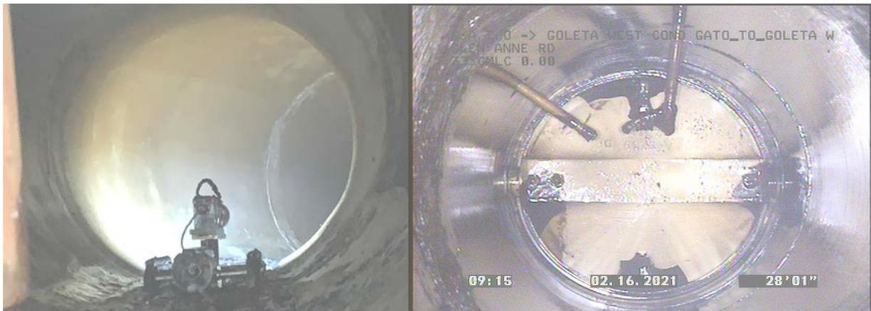
**Figure 3.** Goleta West Conduit – Video Camera Inspection – Inspection camera (left) and bottom of Glen Anne Turnout - Butterfly Valve #5. Mortar lining in good condition and tight seal achieved with Butterfly Valve #5.
