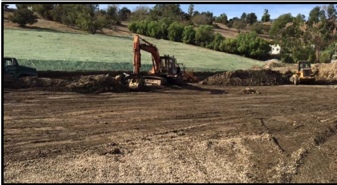
Installation of Geofom over the South Coast Conduit to prevent overloading.
