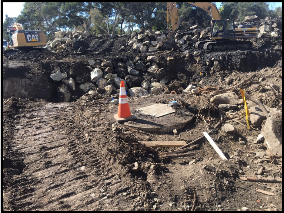
SB County Flood Control Clearing Work at San Ysidro Creek near SCC Crossing
