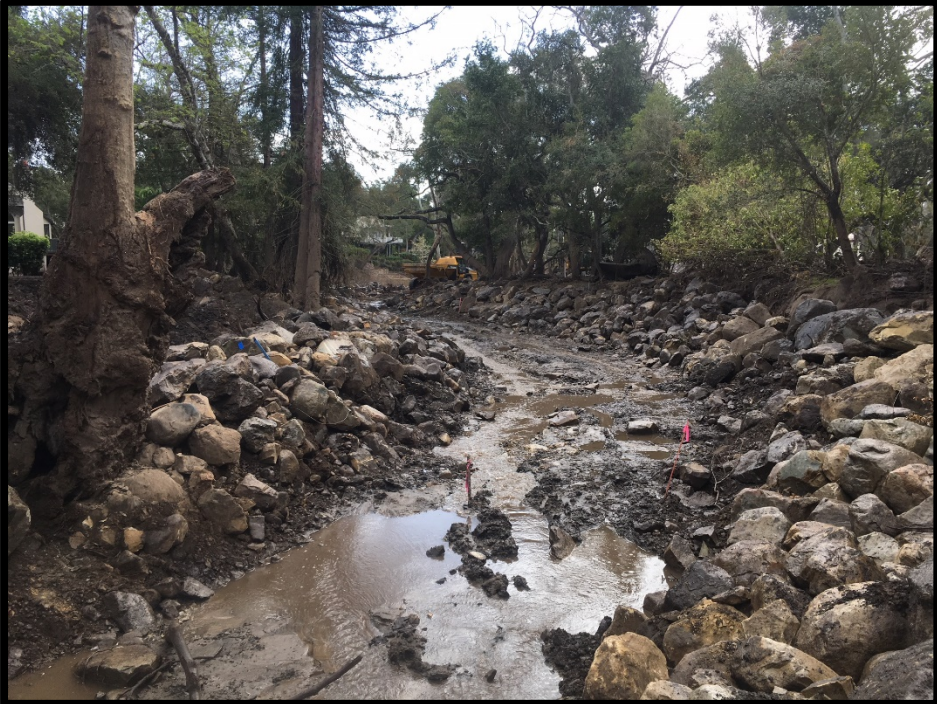
SB County Flood Control Clearing Work at Montecito Creek near SCC Crossing
