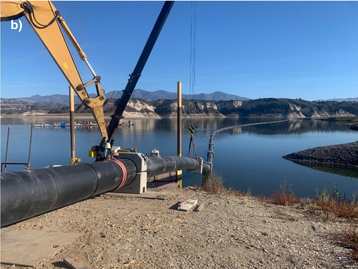
**Figure 5:** a) holdfast installed on end of pipeline; b) 36" by 14" reducing tee for check valve; c) lateral tee installed; d) fully assembled pipeline being towed into position by working barge.
