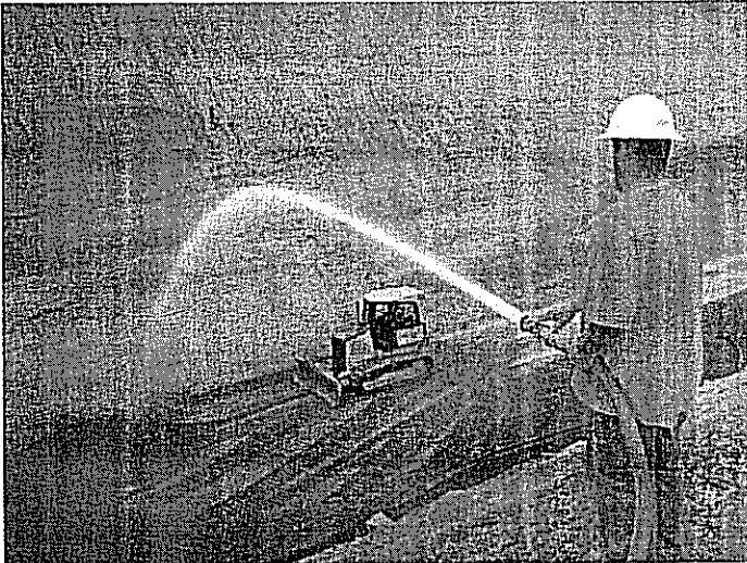
Lauro Dam Construction Project Contractor A.J.Diani Photo by: R. Garcia Date: 5-9-06
