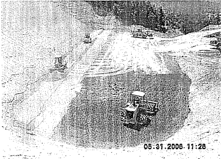
Lauro Dam Construction Project Photo by: L. Campbell
