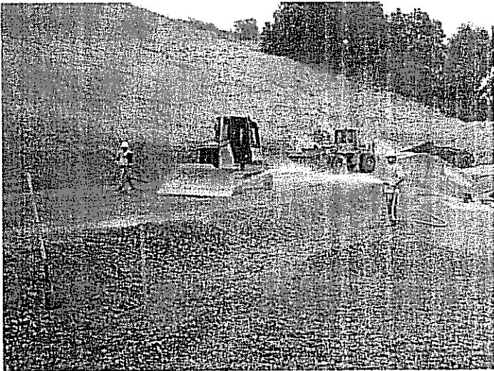
Lauro Dam Construction Project Contractor A.J.Diani Photo by: R. Garcia Date: 5-17-06
