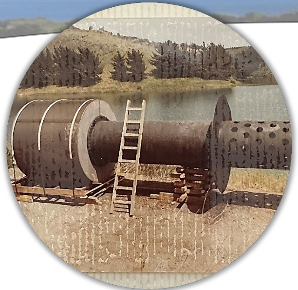
Figure A.6 Intake Structure Extension to be Placed in Lauro Reservoir April 5, 1981
