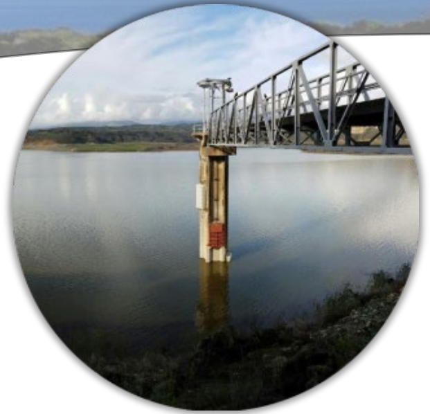
Figure A.10 North Portal Intake Tower
