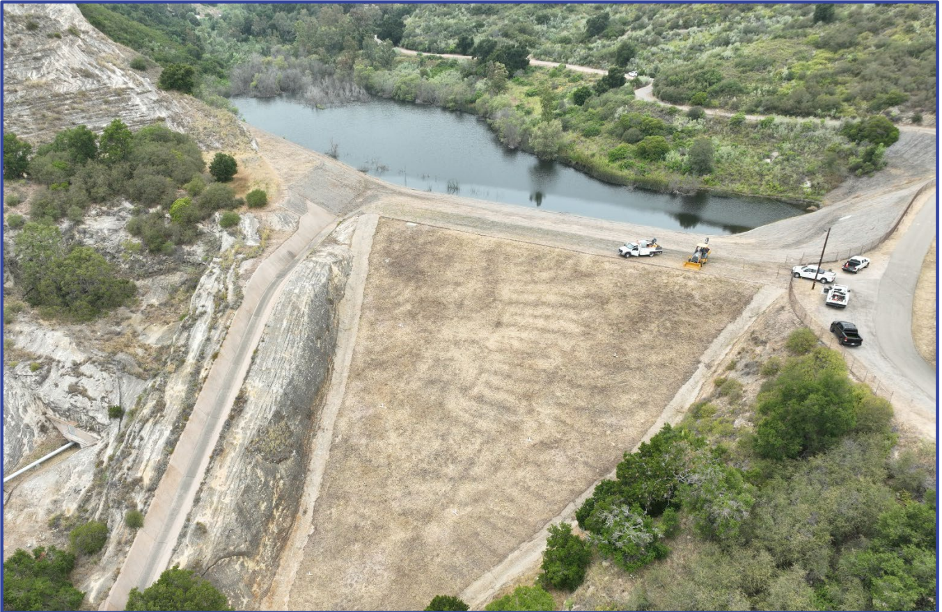
Figure 2. Glen Anne Dam and Reservoir Maintenance Activities
