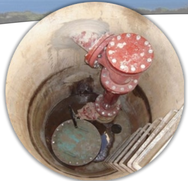
Figure A.3 Inside of Blowoff Structure
