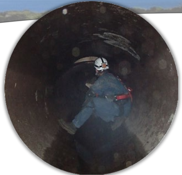
Figure A.11 Previous Inspection of SCC Interior
