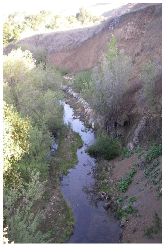
Figure 6-13. El Jaro Creek Demonstration Project: Stabilization of eroding streambank
