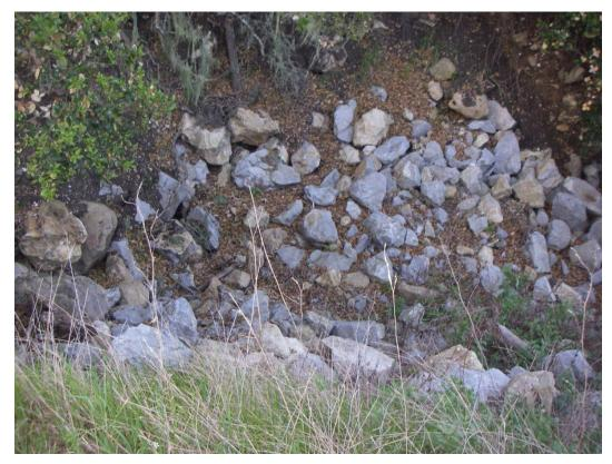
Figure 6-12. El Jaro Creek Demonstration Project: Stabilization of exposed side draw
