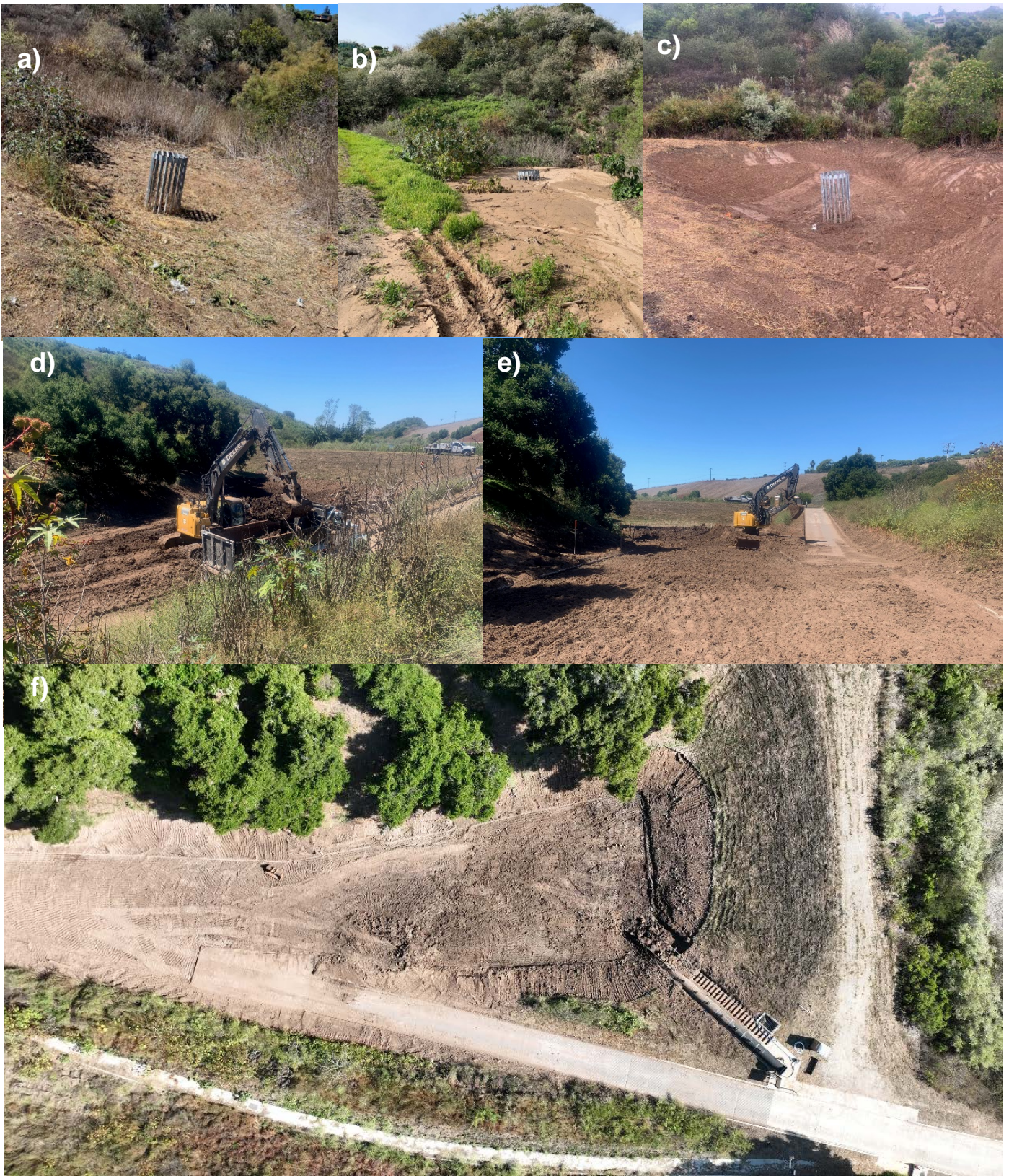
Figure 1. Clearing of sediment from San Roque Road Basin a) before storm; b) post-storm; c) post cleanup and Lauro Main Debris Basin clearing (d,e,f)
