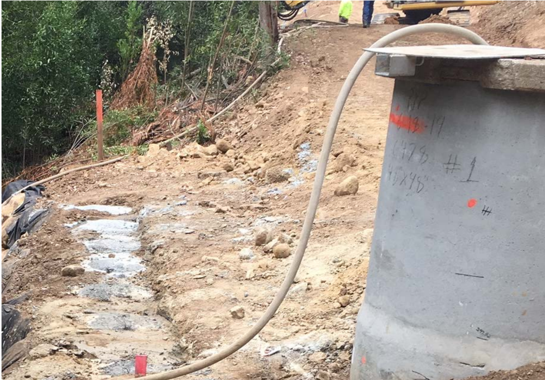
Middle wall reinforced caissons completed
