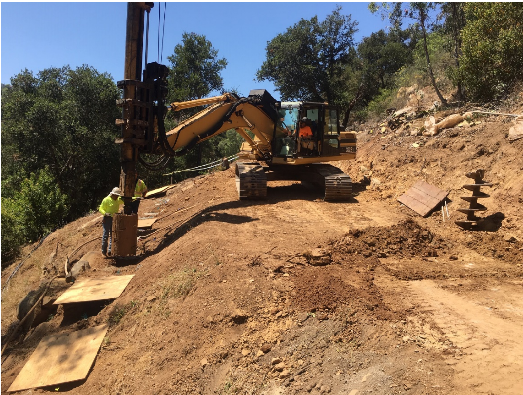
Drilling hole for reinforced caisson with a core bucket
