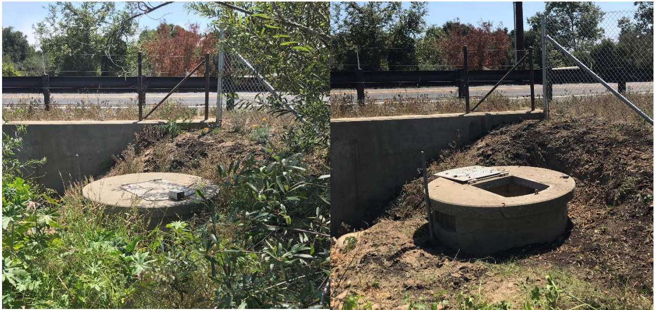
Cleared vegetation from structure 698+55
