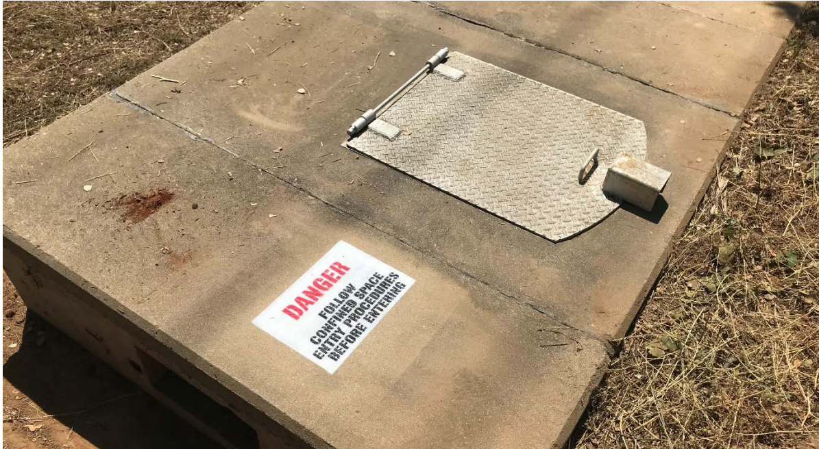
Repainting warning sign on structure 691+50
