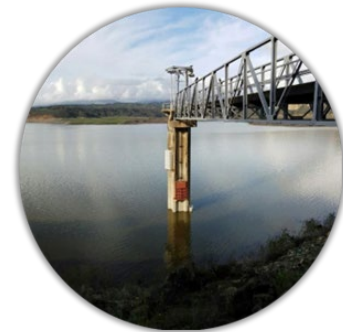
Figure - North Portal Intake Tower
