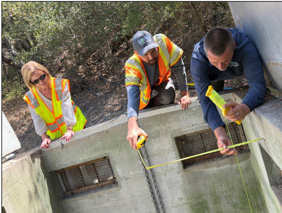
Sheffield Tunnel East Portal
