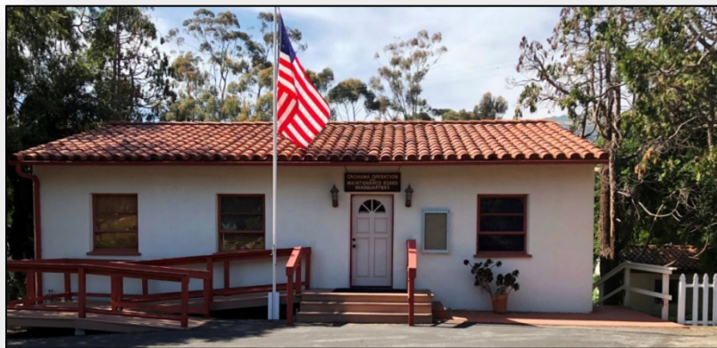
Cachuma Operation and Maintenance Board Meeting Room
