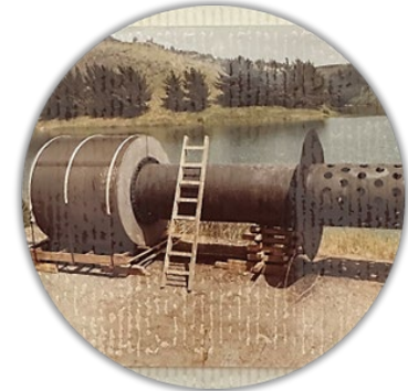
Figure - Intake Structure Extension to be Placed in Lauro Reservoir April 5, 1981
