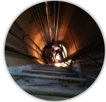
Figure - North Portal Elevator Shaft
