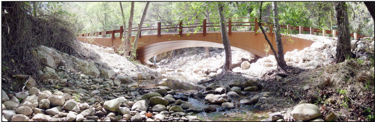
Quiota Creek Fish Passage Project
