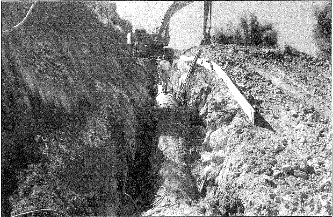
Laying Pipe, Placing Sand Backfill and Constructing Trench Cutoff Wall
