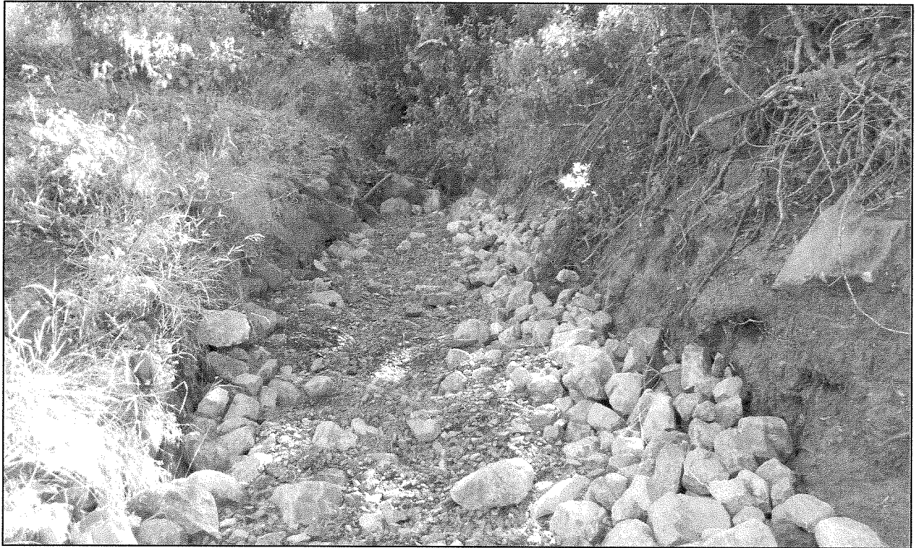
Restored Stream Bed
