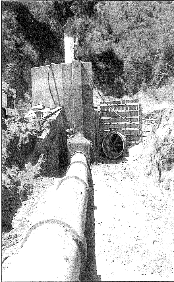
Overflow Drain at Junction Structure Prior to Relocation
