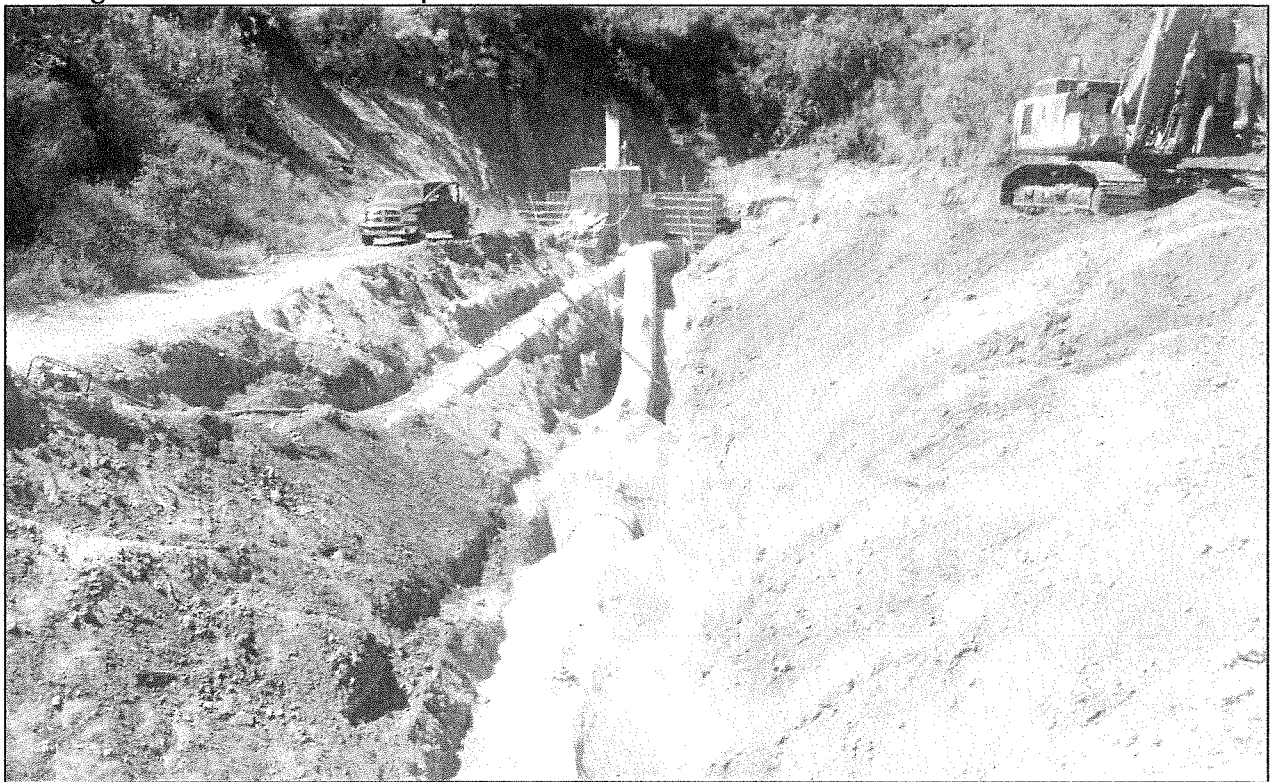
Relocated Overflow Drain and New SSC
