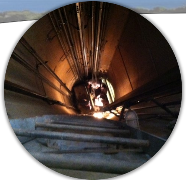
Figure A.1 North Portal Elevator Shaft
