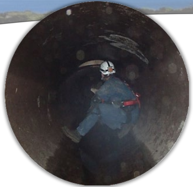
Figure A.11 Previous Inspection of SCC Interior
