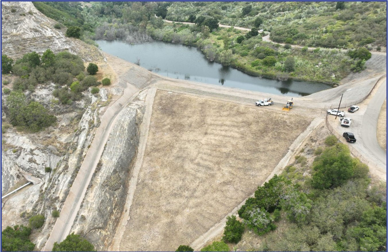
Figure 2. Glen Anne Dam and Reservoir Maintenance Activities
