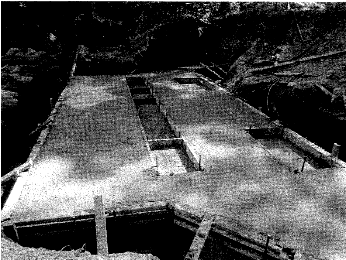
Figure 8: Pouring the bridge foundations (9/17/12).
