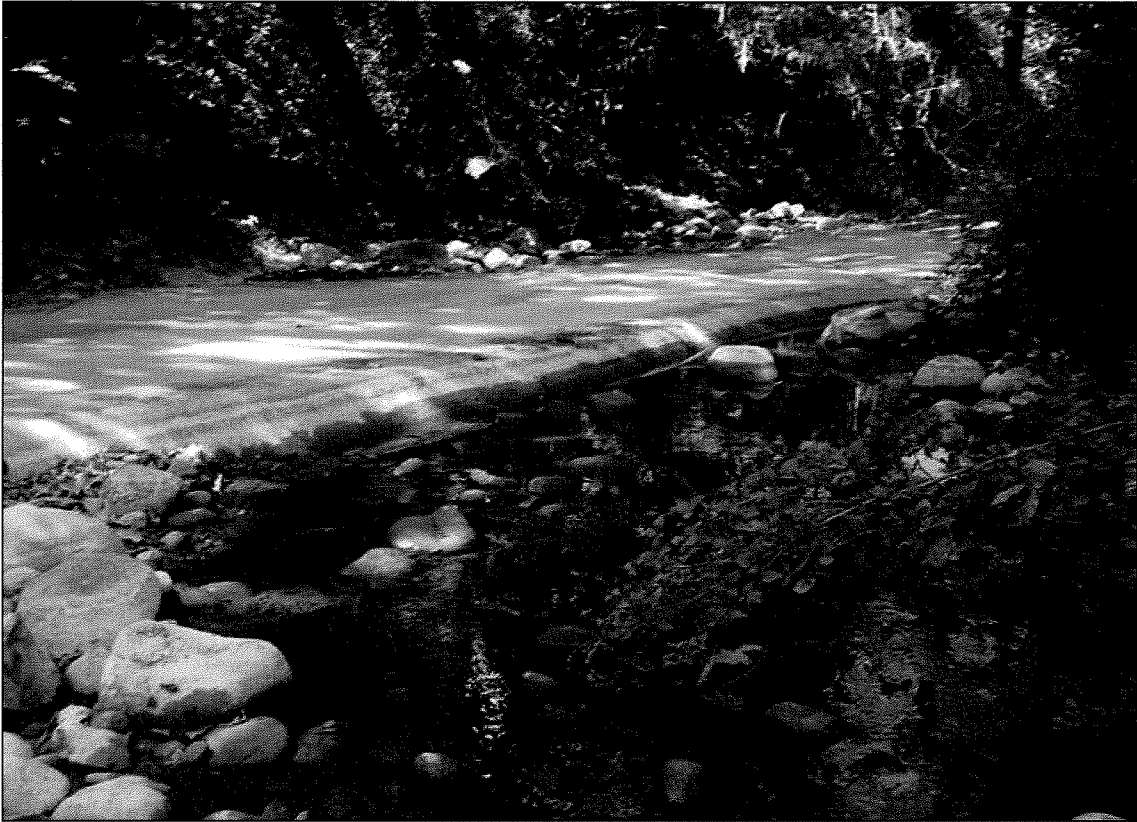
Figure 1: Quiota Creek Crossing 7, pre-project condition.
