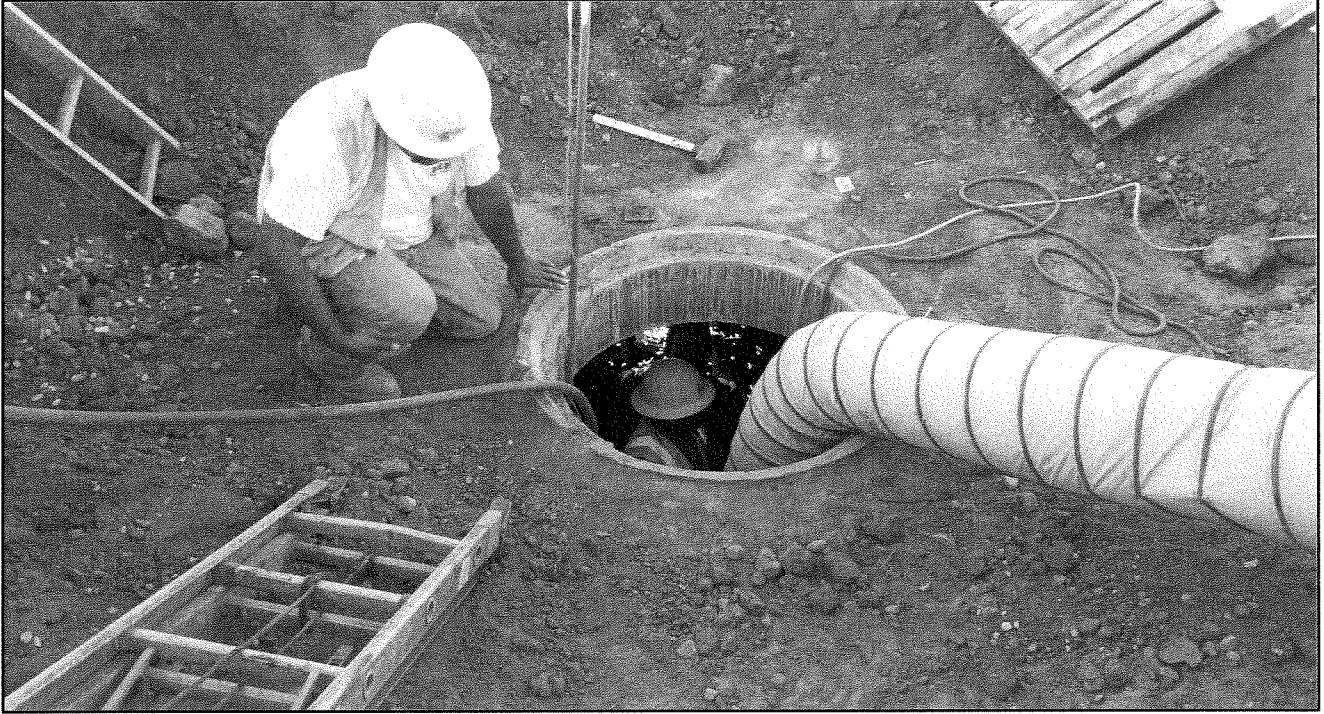
Working in Goleta West Meter Vault during shutdown
