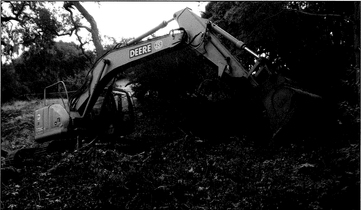
Figure 4: Clearing and grubbing (9/5/12).
