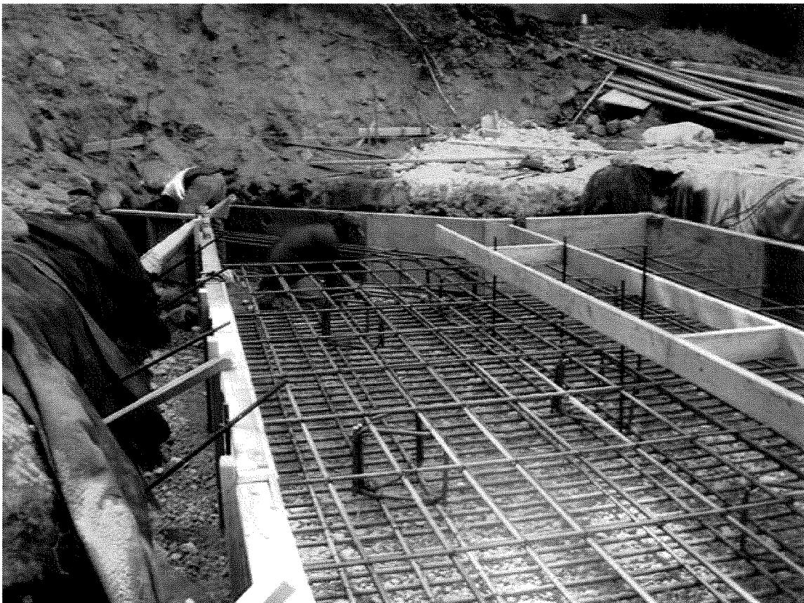
Figure 6: Bridge footing preparation (9/14/12).
