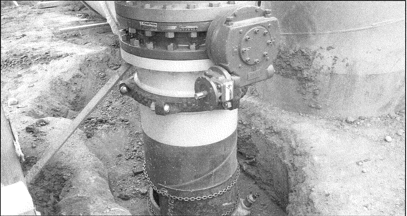
Fitting up connection between new 48" pipe and existing Goleta West Pipe
