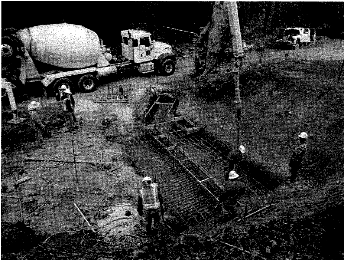
Figure 7: Pouring the bridge foundations (9/17/12).
