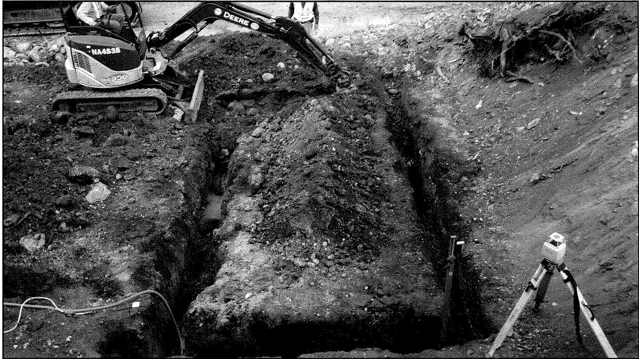
Figure 5: Excavating footing for bridge abutment (9/10/12).
