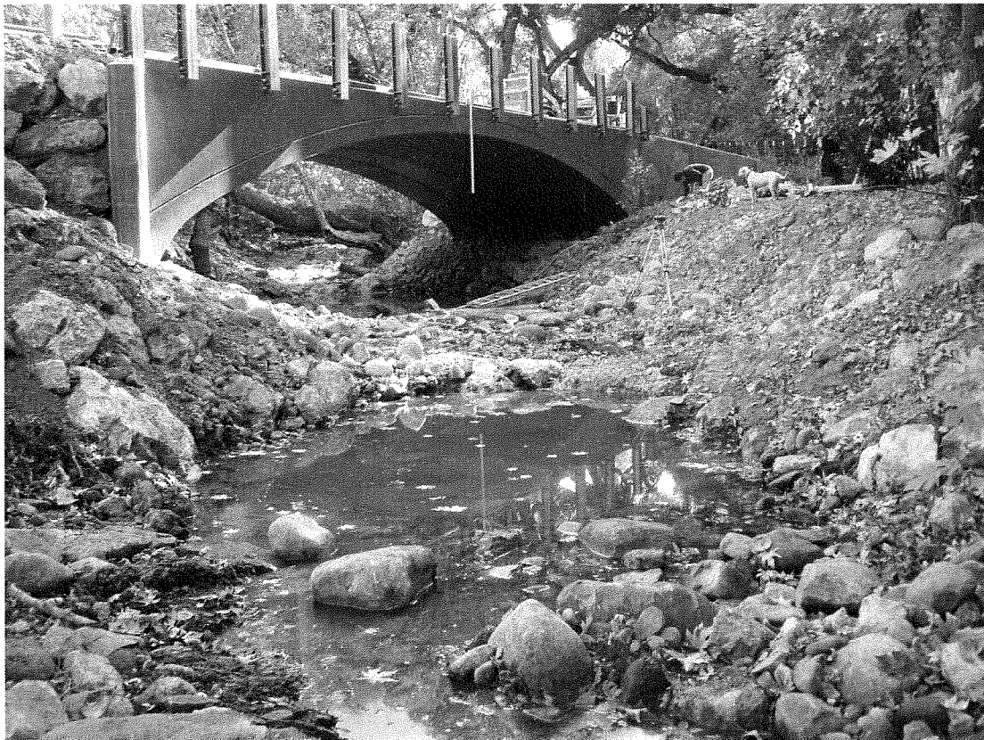
Figure 6: All stream work completed, view looking upstream (11/14/12).
