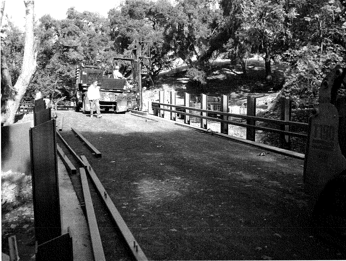
Figure 11: Bridge-rail installation (11/14/12).
