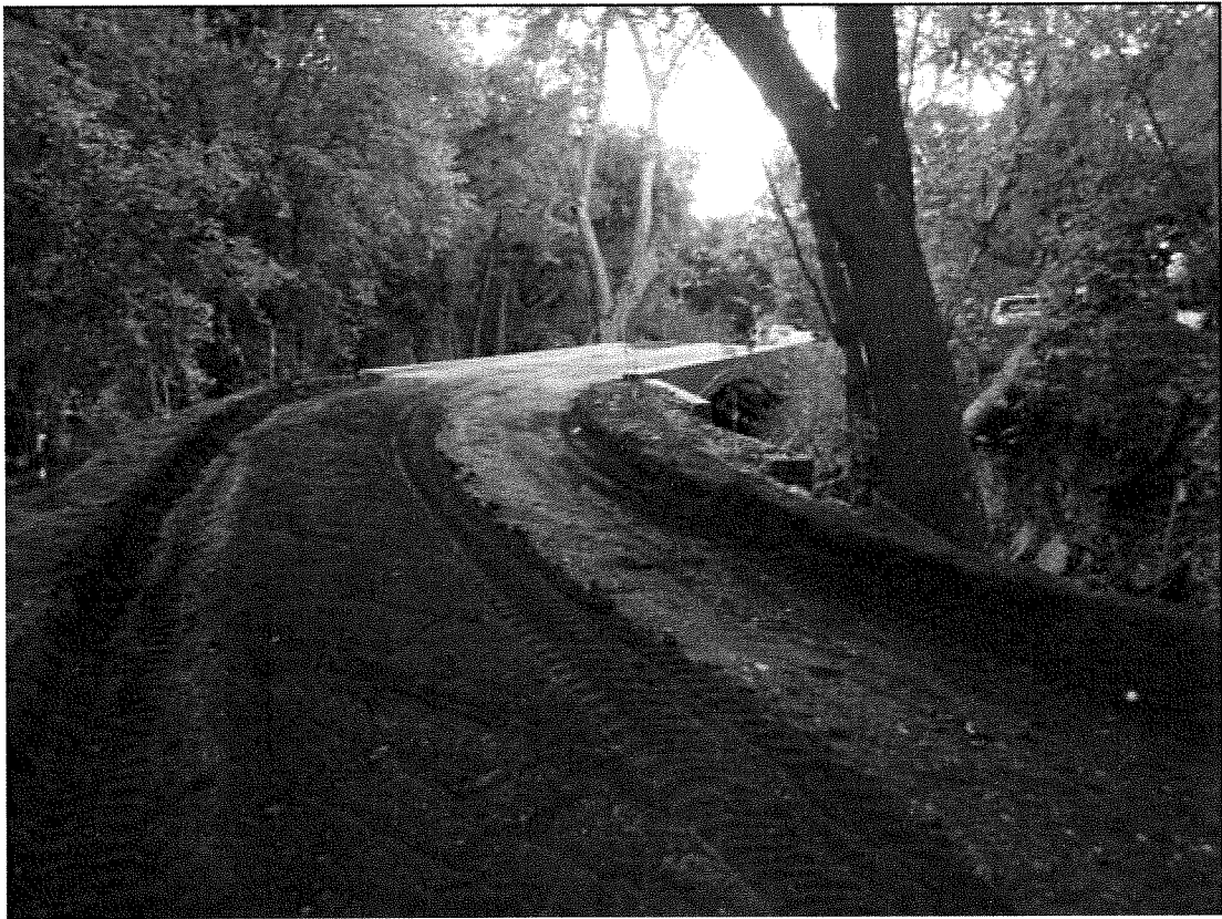
Figure 4: Road base preparation (10/29/12).
