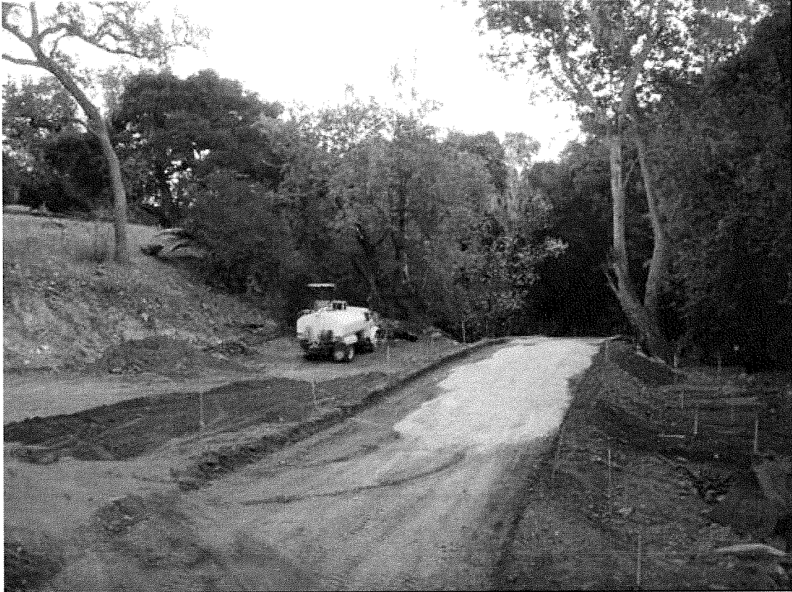
Figure 3: Road base preparation (10/29/12).
