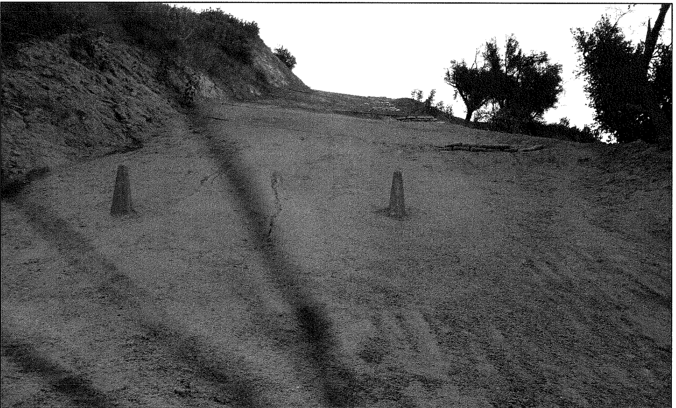
Hydroseeded Slope
