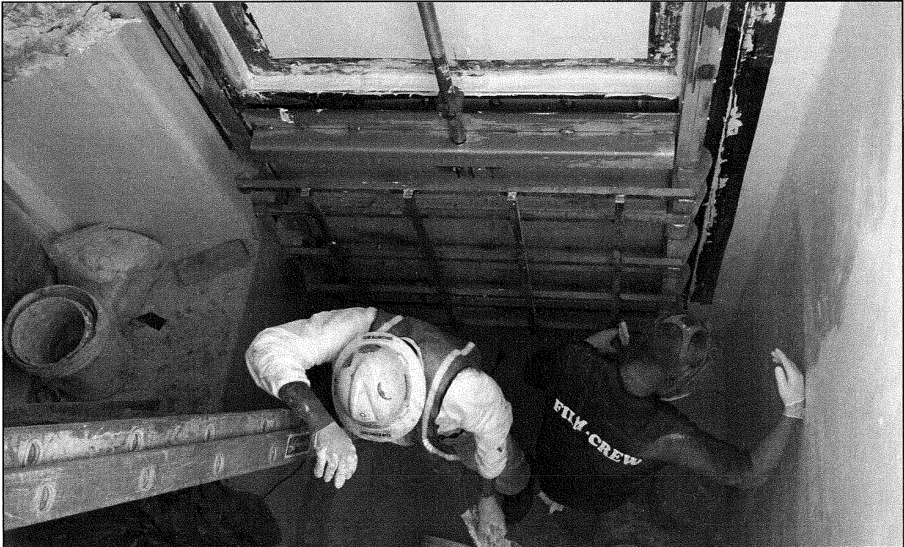
installing slide gate
