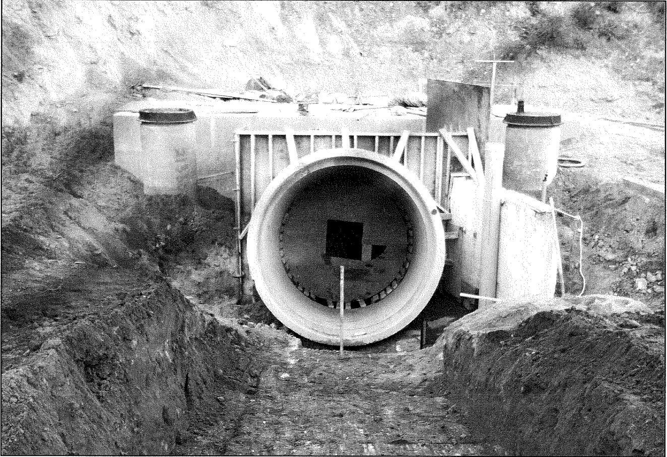
New 84" Tunnel Access
