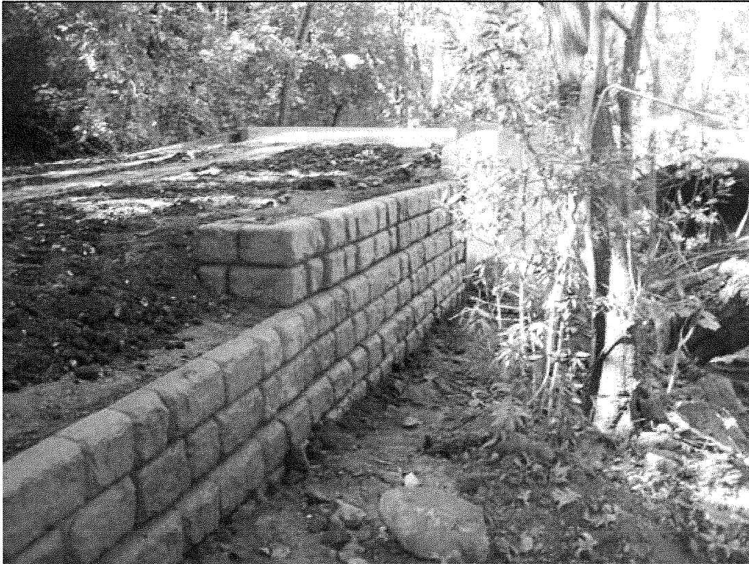
Figure 5: Ready-Rock Wall installed (10/26/12).
