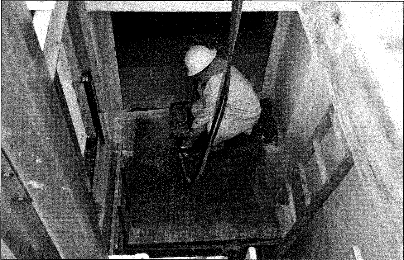
Saw cutting South Portal Junction Structure walls with diamond blade
