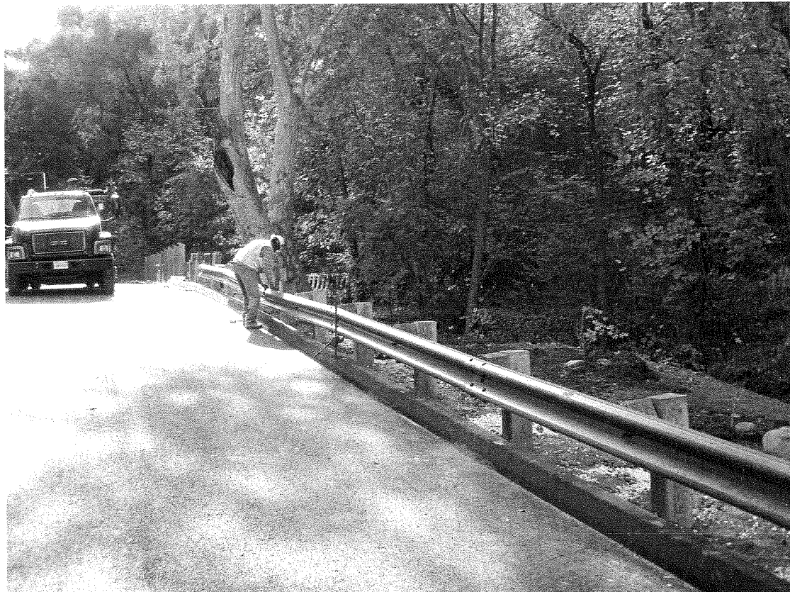
Figure 12: Guardrail installation (11/14/12).
