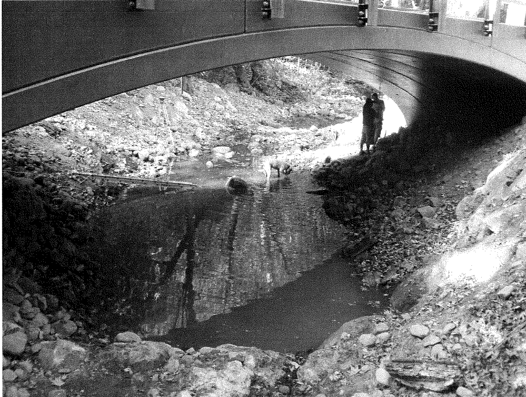
Figure 7: All stream work completed, view looking downstream (11/14/12).
