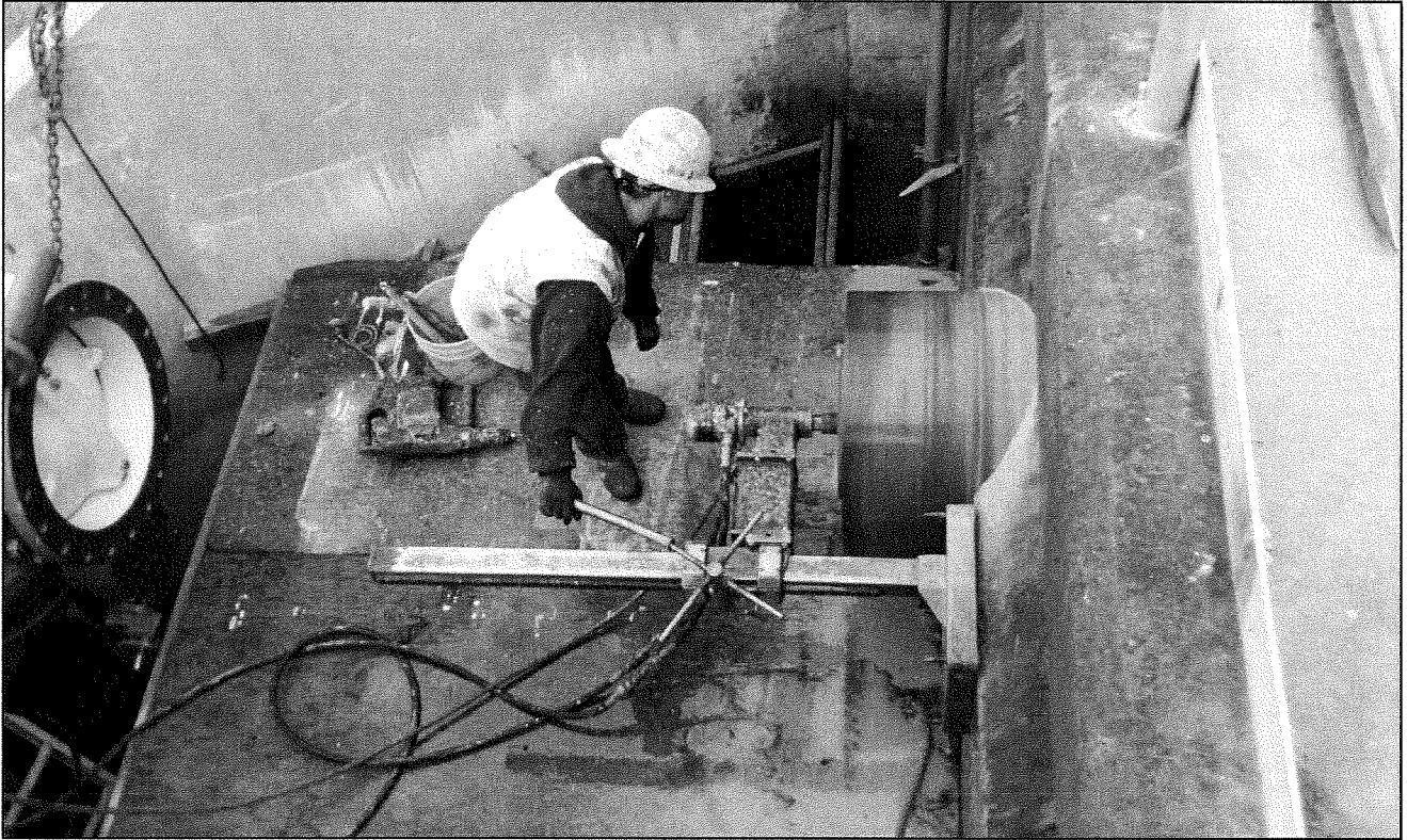
Cutting hole into GATO structure for 24" drain pipe
