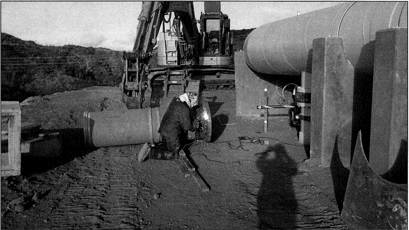
Welding flange on pipe
