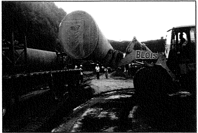
Unloading pipe. Only 2-40' long sections can be carried on a truck
