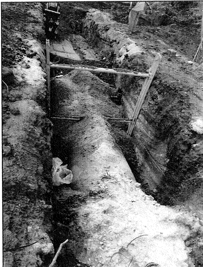
Placing sand backfill in pipe zone
