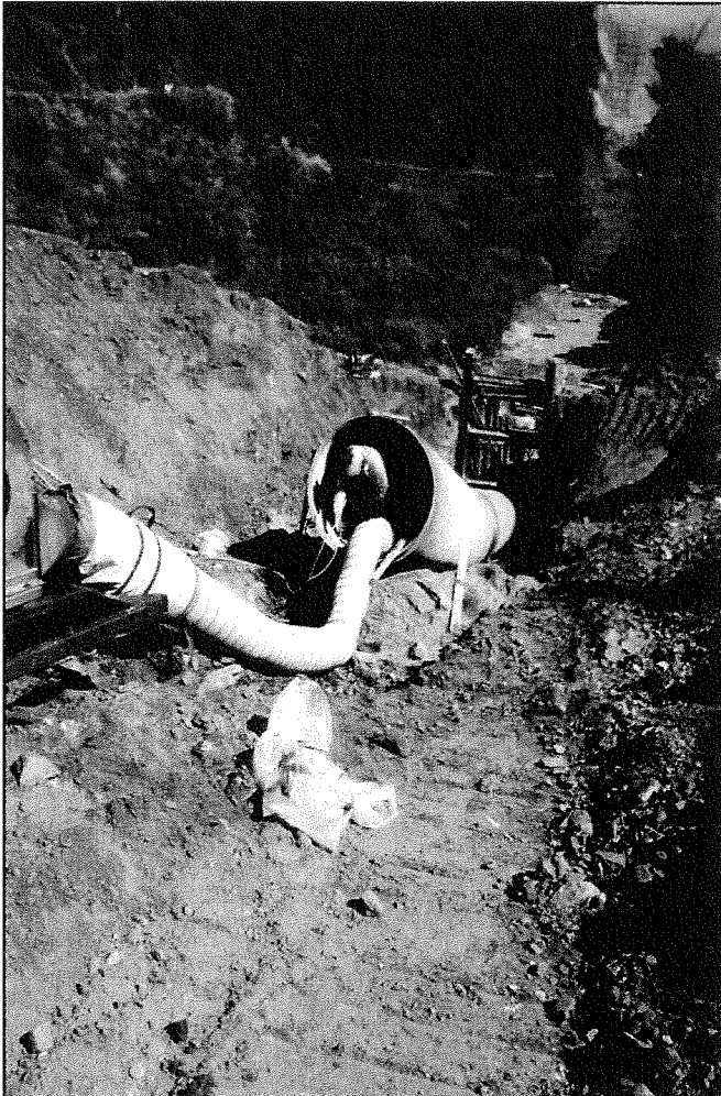
Blower being used to ventilate pipe while welder is inside pipe
