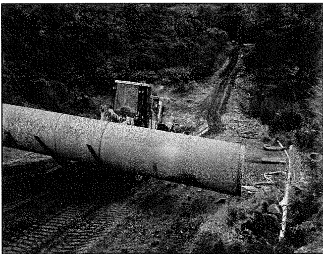
Pipe section being carried to bottom of slope
