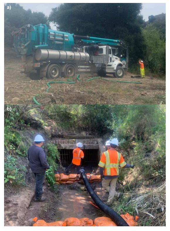
**Figure 2**. Lauro Reservoir Spillway Stilling Well (a) combination hydrojetting vacuum truck utilized to remove debris; (b) 300 feet of 6-in corrugated HDPE pipe utilized to transport vacuumed sediment and water and sandbag dams utilized to contain the sediment.
