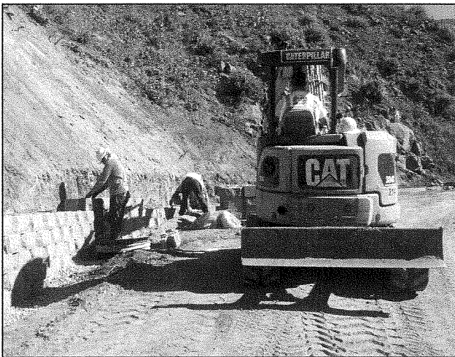
Constructing Gravity Wall on GATO Access Road
