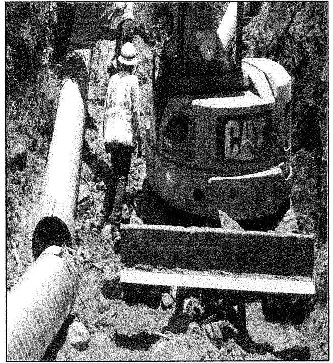
Extending Storm Drain
