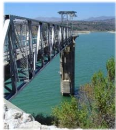
Intake Tower at Lake Cachuma
