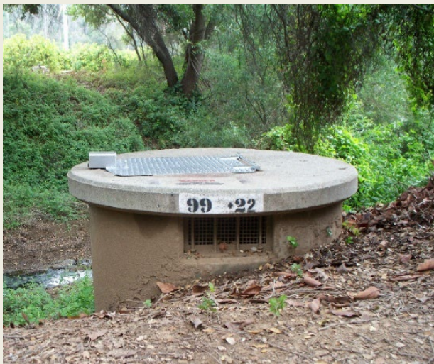
Figure 7. Blowoff Structure at Station 99+22
