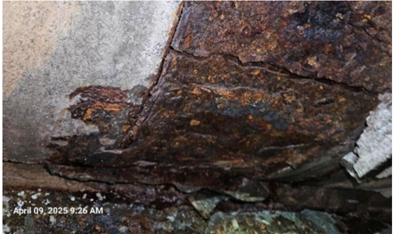
Figure 4. Examples from the April 2025 inspection of the Sheffield Tunnel showing exterior mortar and metal joint ring damage at the pipe joint.
