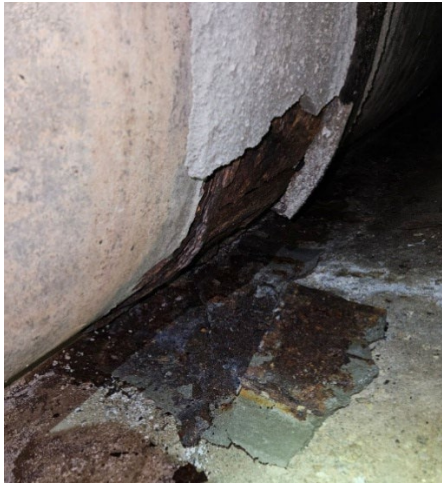
Figure 4. Examples from the April 2025 inspection of the Sheffield Tunnel showing exterior mortar and metal joint ring damage at the pipe joint.
