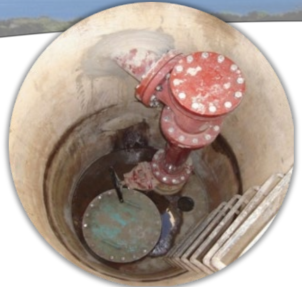
Figure A.3 Inside of Blowoff Structure
