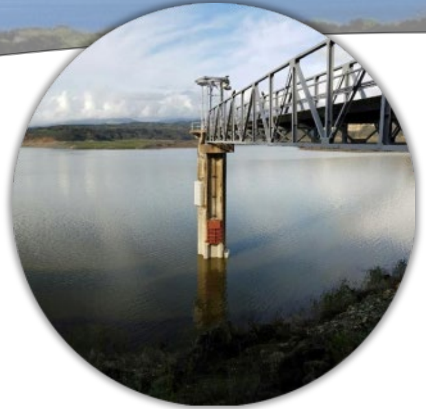
Figure A.10 North Portal Intake Tower
