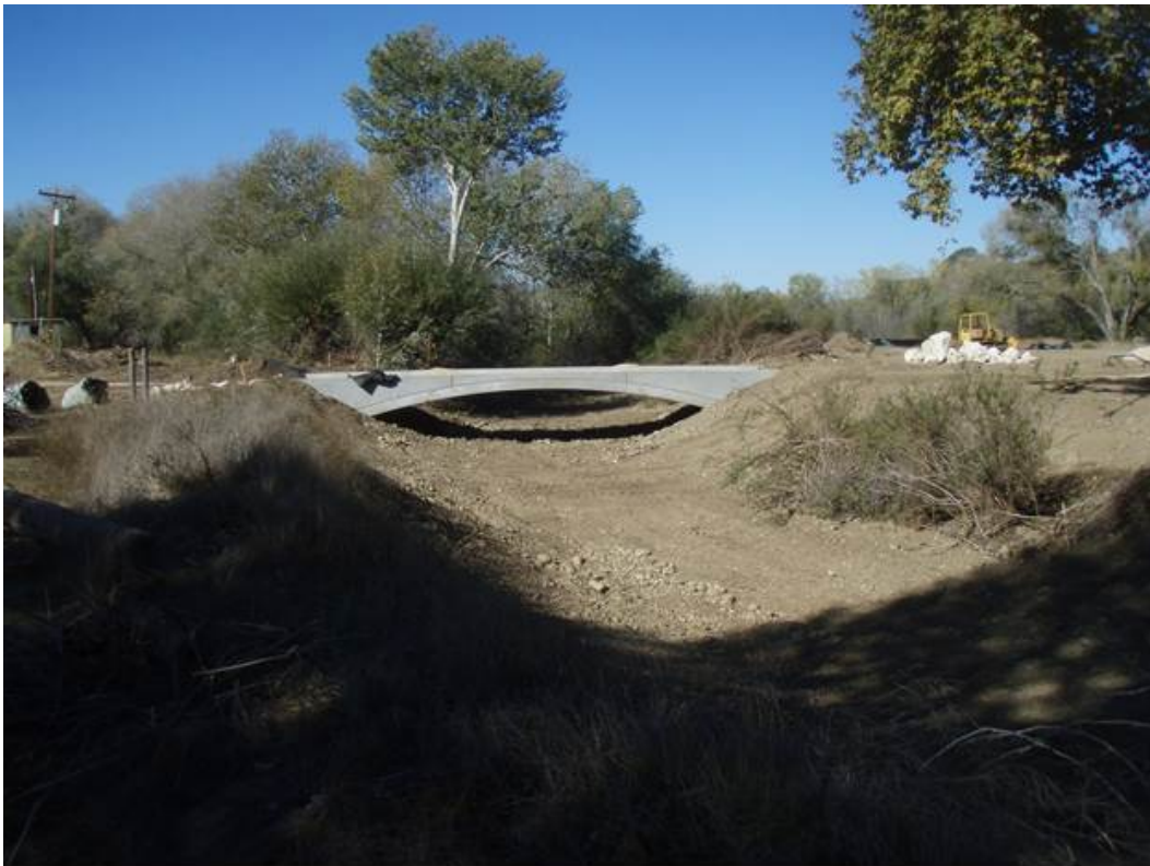
Figure 7: Completed stream work.
