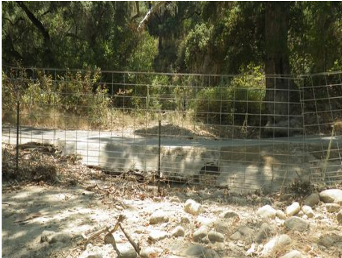
Figure 1: Pre-project condition looking upstream.
