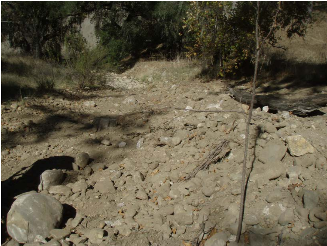
Figure 6: Stream work, toe of slope rocks downstream of the bridge.
