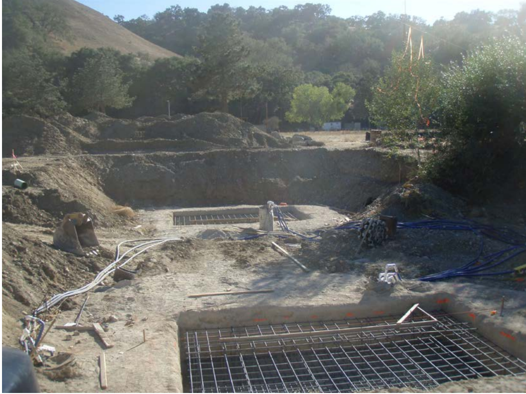
Figure 2: Bridge foundation construction.
