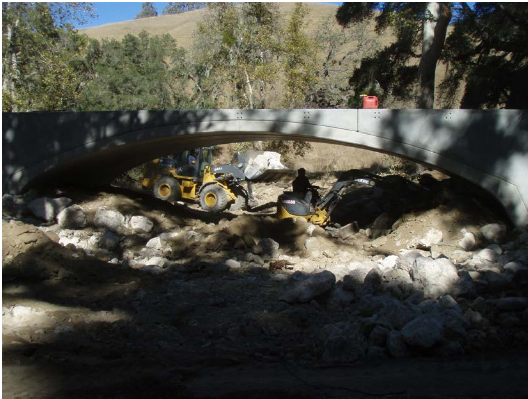
Figure 5: Rock slope protection installation.
