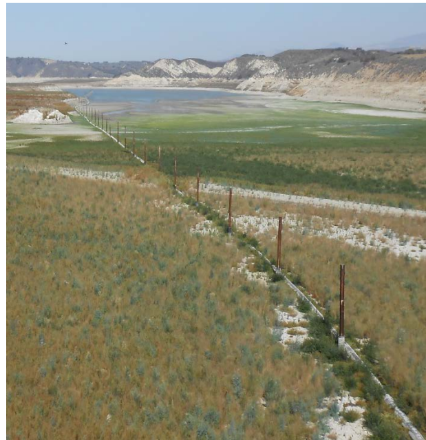
Figure 2. Mooring of existing pipeline using steel piles. Piles are spaced at 100 feet. Photo on left was taken when the barge was at Site 1 and the lake was approximately 20 percent full. Photo on right shows the same view in September 2016, with the lake at 7 percent full and the barge moved down the lake to Site 2.
