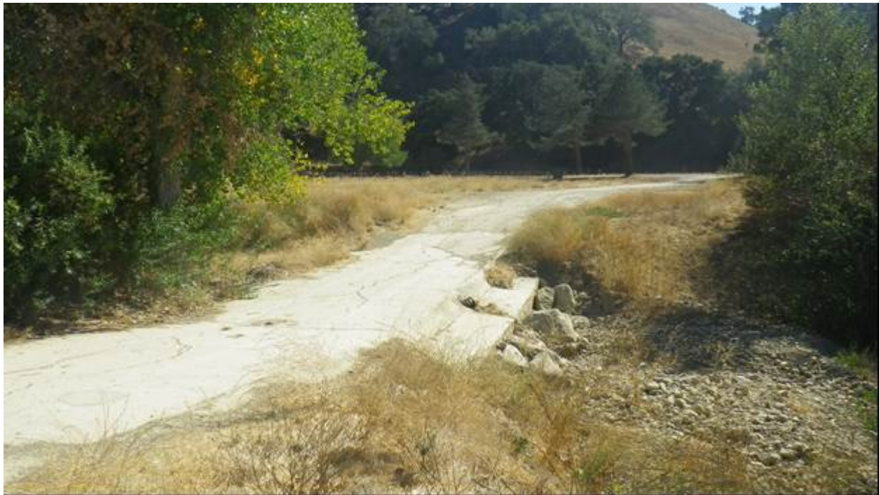
Figure 1: Pre-project condition looking upstream.
