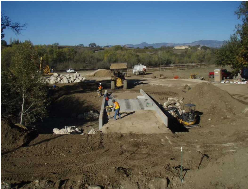
Figure 5: Back filling of the arch.
