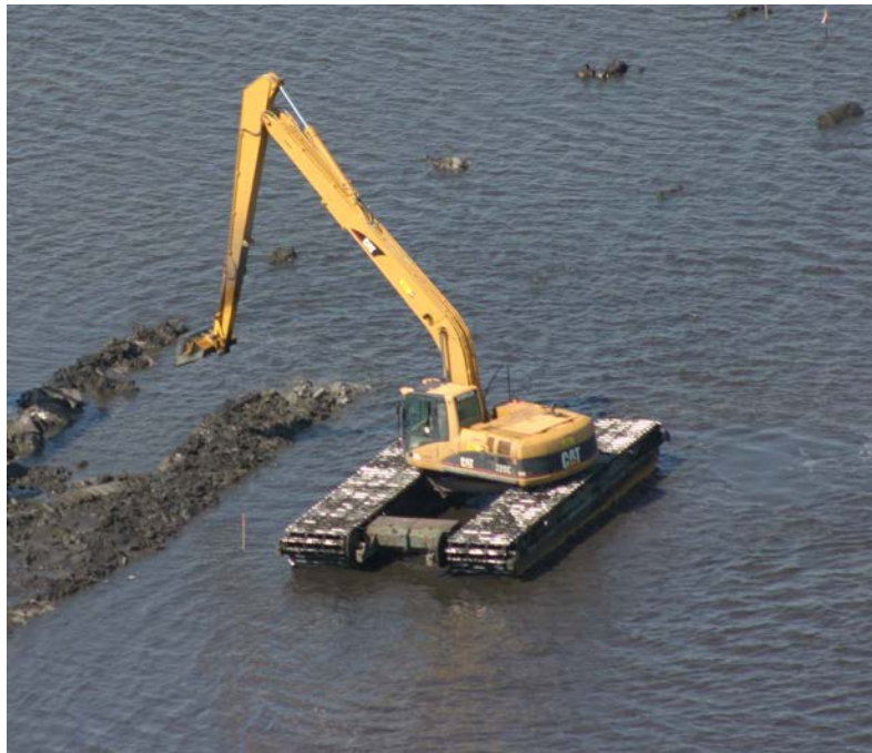
Figure 6. Example of Amphibious Construction Equipment. Equipment like this is needed where water is too shallow for barges and land is too soft for conventional tracked equipment.
