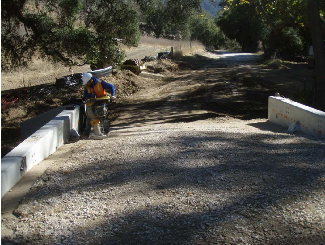
Figure 8: Backfilling of the arches with road compaction.
