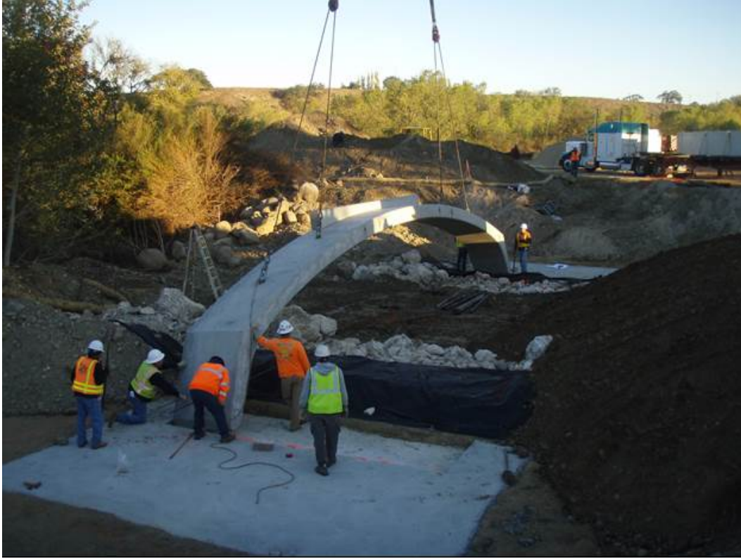
Figure 4: Bridge installation.
