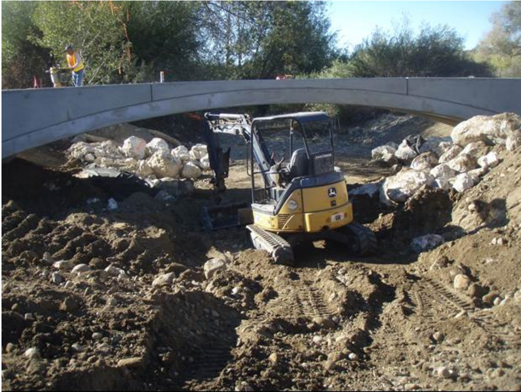
Figure 6: Installation of the rock slope protection.
