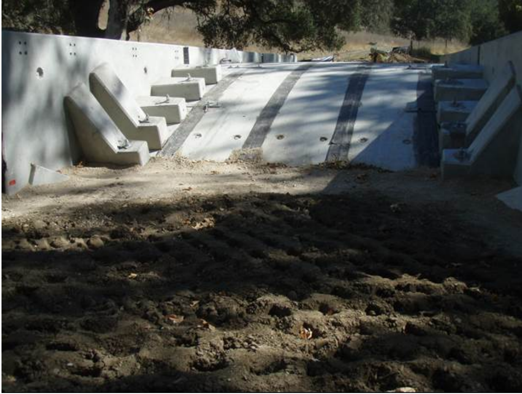
Figure 4: Backfilling the arched bridge.
