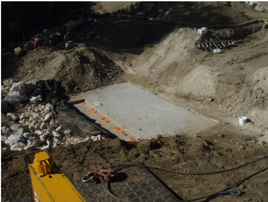
Figure 3: Completed bridge foundations.
