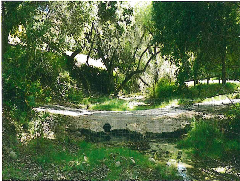
Figure 2: Quiota Creek on Refugio Road showing side-view of Crossing 3.
