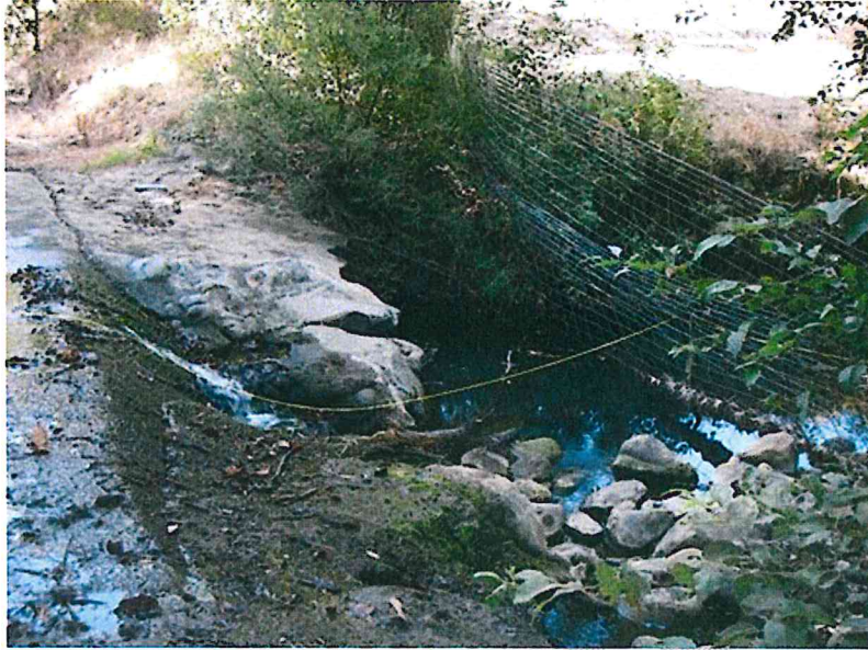
Figure 7: Quiota Creek on Refugio Road showing side-view of Crossing 9.
