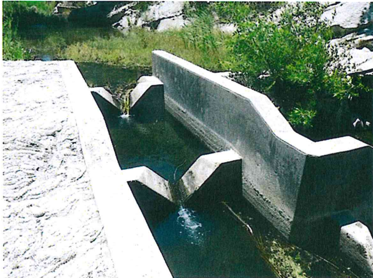
Figure 5: Salsipuedes Creek fish ladder at Jalama Road showing weirs that need to be fixed.
