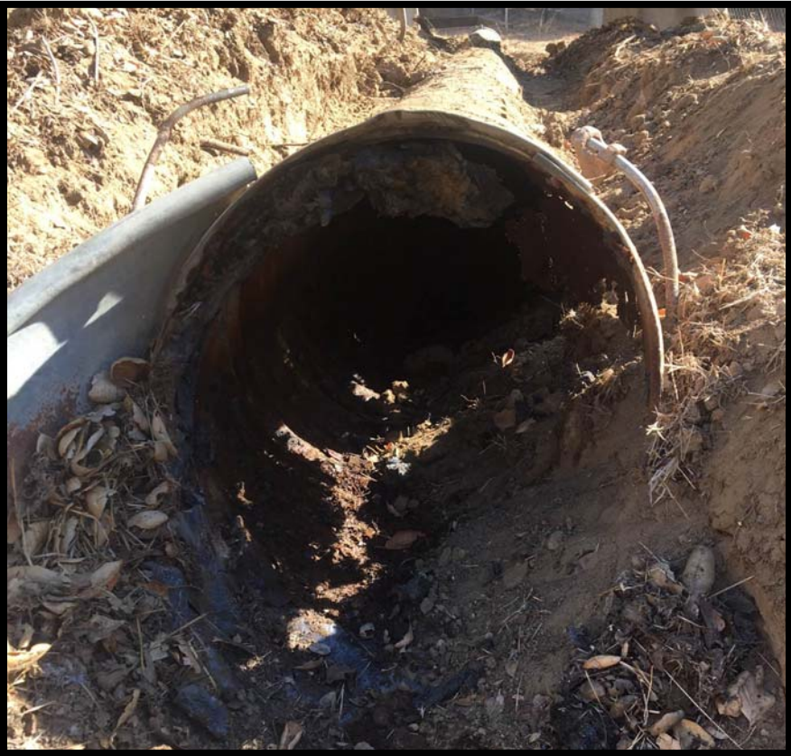
Original Corroded Pipe
