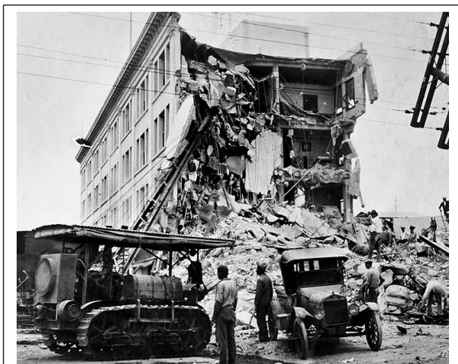
Damage from the 1925 Santa Barbara earthquake
