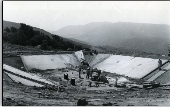
Construction of Bradbury Dam
