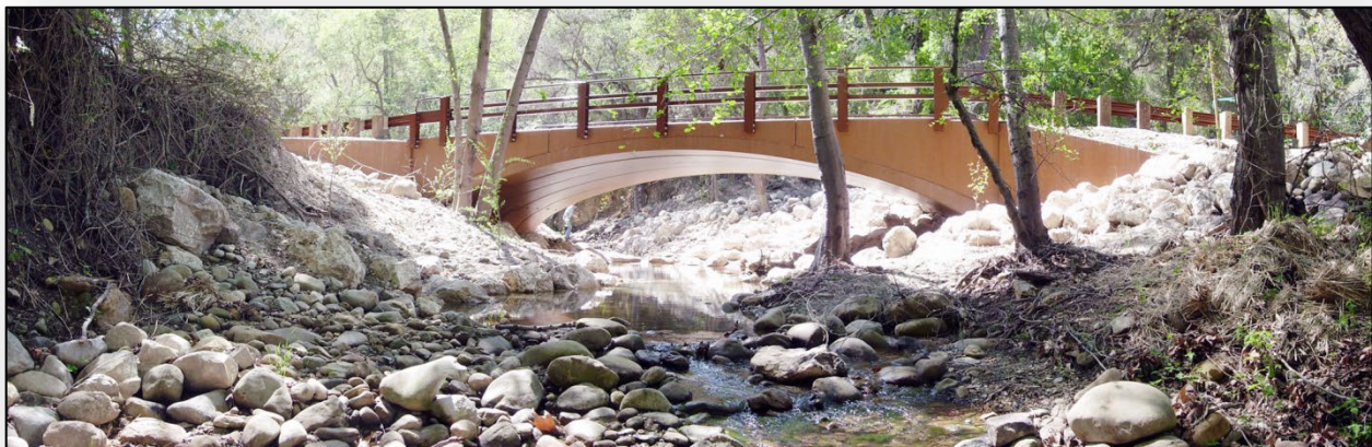
Quiota Creek Fish Passage Project
