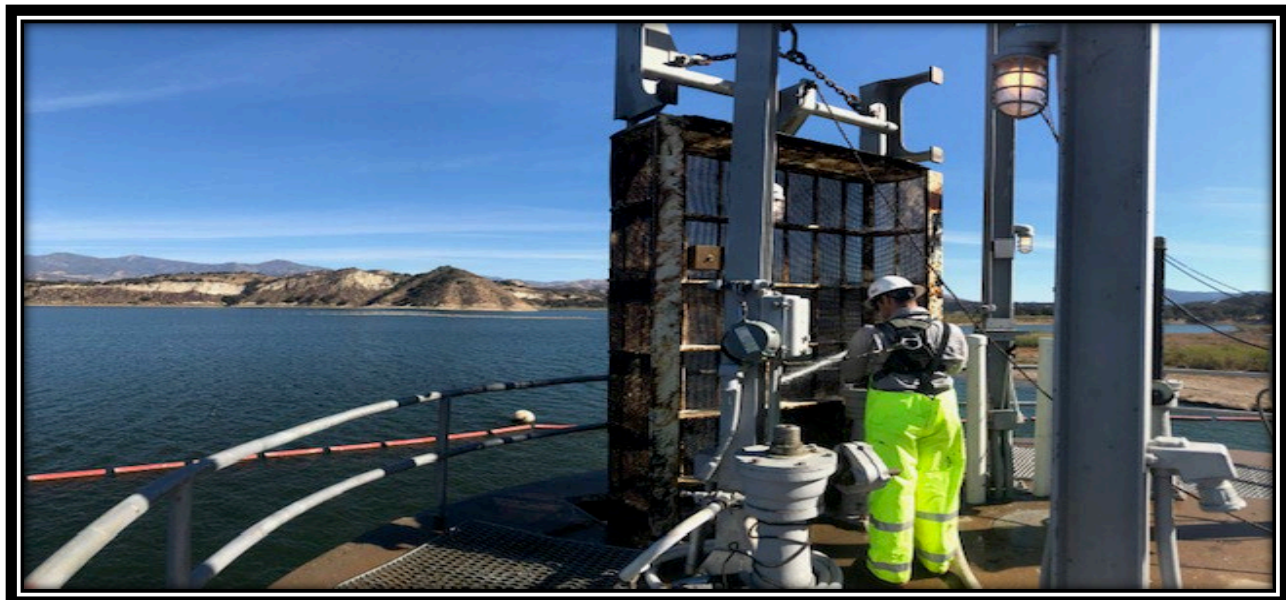
North Portal Intake Tower
