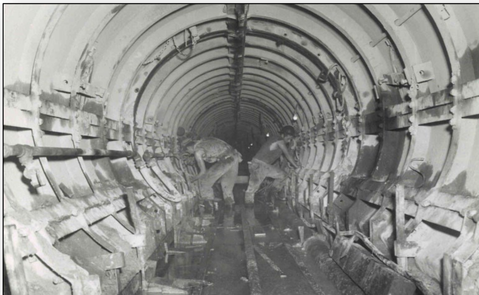
Tecolote Tunnel Construction
