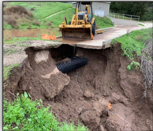
Lauro Reservoir Access Road
