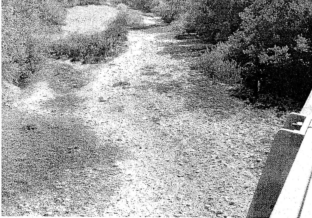
Highway 154 Bridge Looking Upstream, Thursday Sept. 4, 2003
