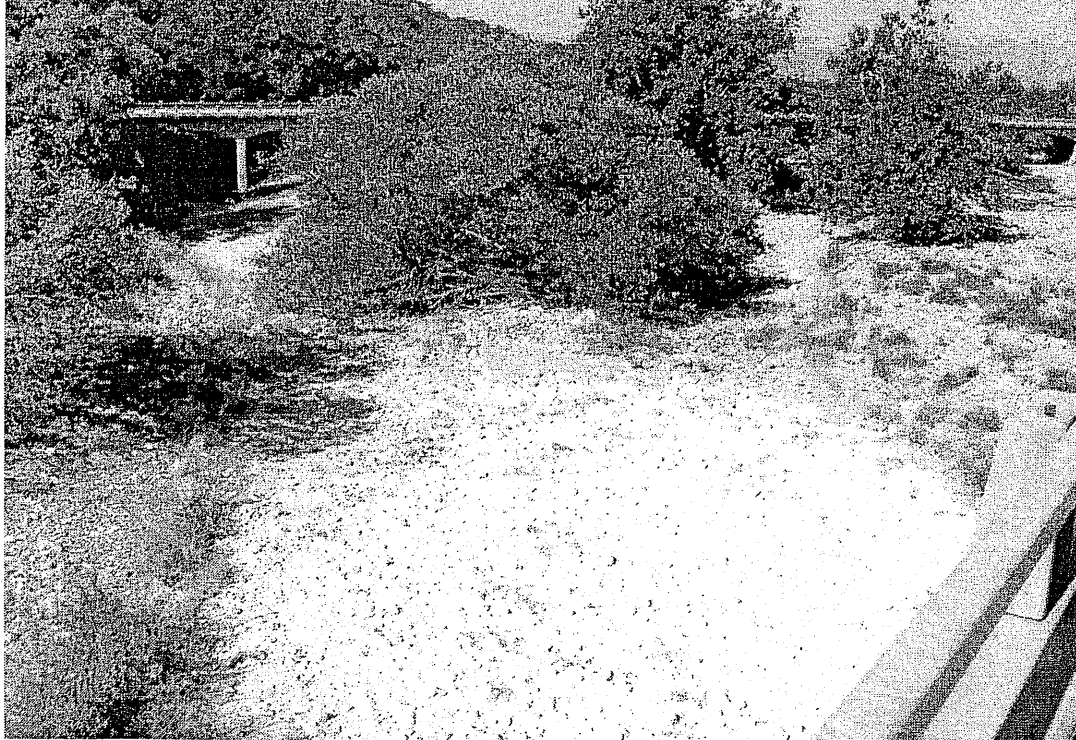
Highway 154 Bridge Looking Downstream, Thursday, Sept. 4, 2003
