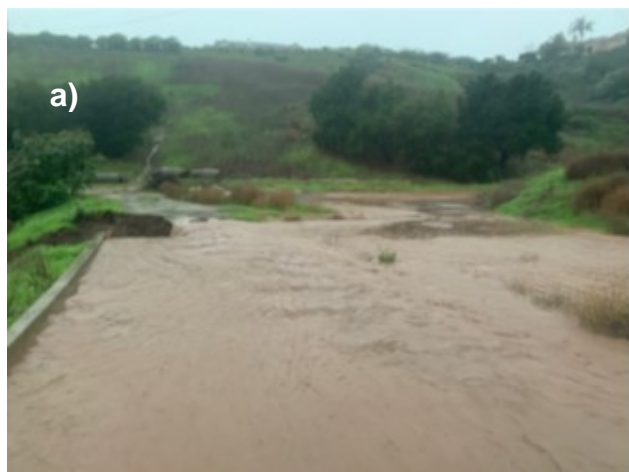
Figure 2. Lauro Reservoir Bypass Channel/Road (a) washout during the January 9, 2023 event and (b) repaired, improved, and tested during the December 21, 2023 storm event.
