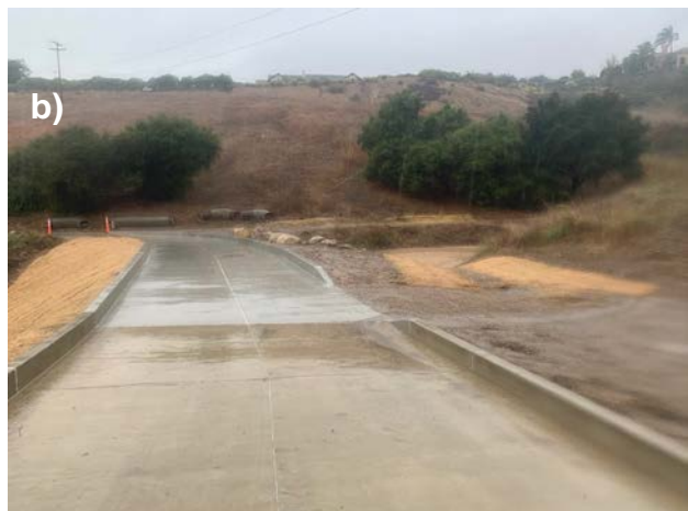
Figure 2. Lauro Reservoir Bypass Channel/Road (a) washout during the January 9, 2023 event and (b) repaired, improved, and tested during the December 21, 2023 storm event.
