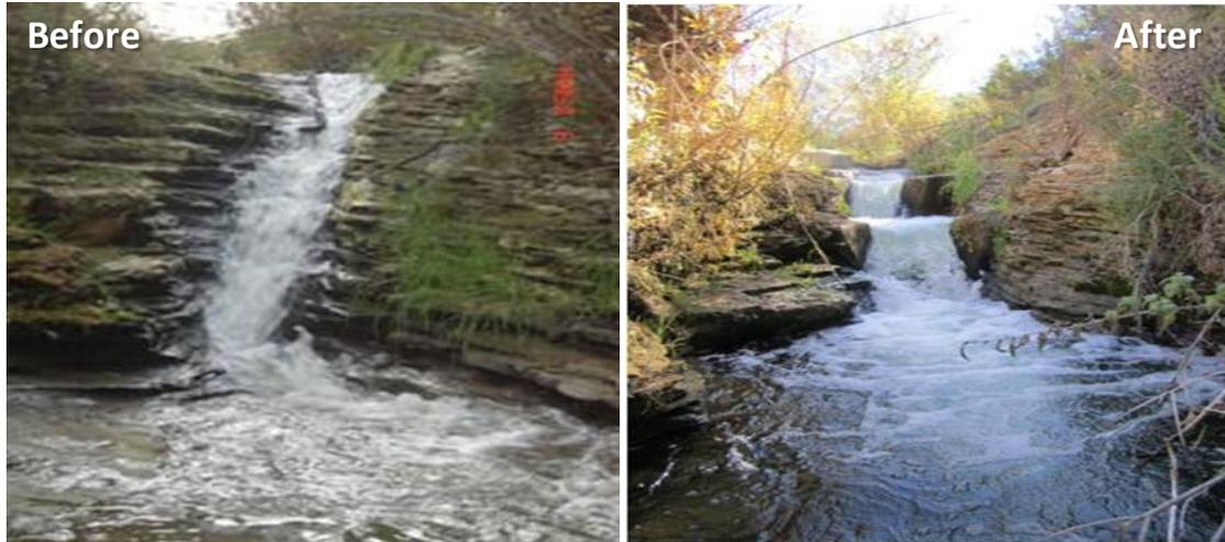
**Figure 78:** Fish passage and habitat restoration at Hilton Creek at the Cascade Chute Project that was completed in 2005.
