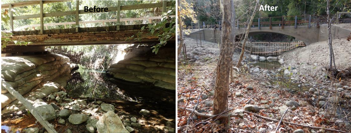
Figure 116: Fish passage and habitat restoration at Quiota Creek Crossing 8 completed in 2019.
