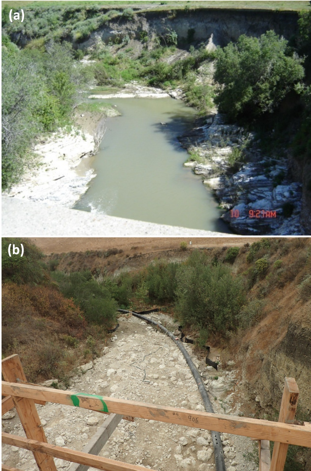
Figure 65: Photo point (T-39) collected at Salsipuedes Creek at Hwy 1 Bridge in May 2005 and (b) September 2020 (during Caltrans bridge replacement project).
