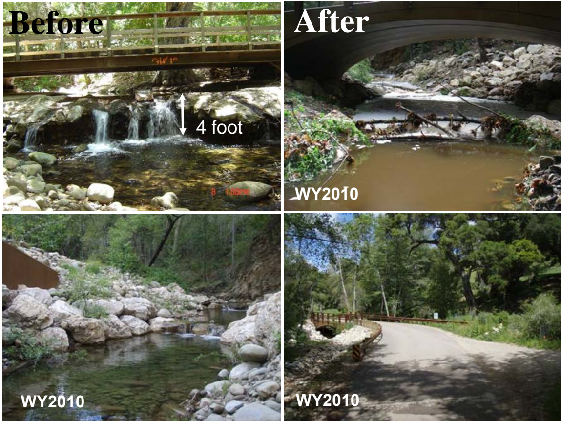
Figure 51: Fish passage and habitat restoration in the fall of 2008 at Refugio Road on Quiota Creek Crossing 6.
