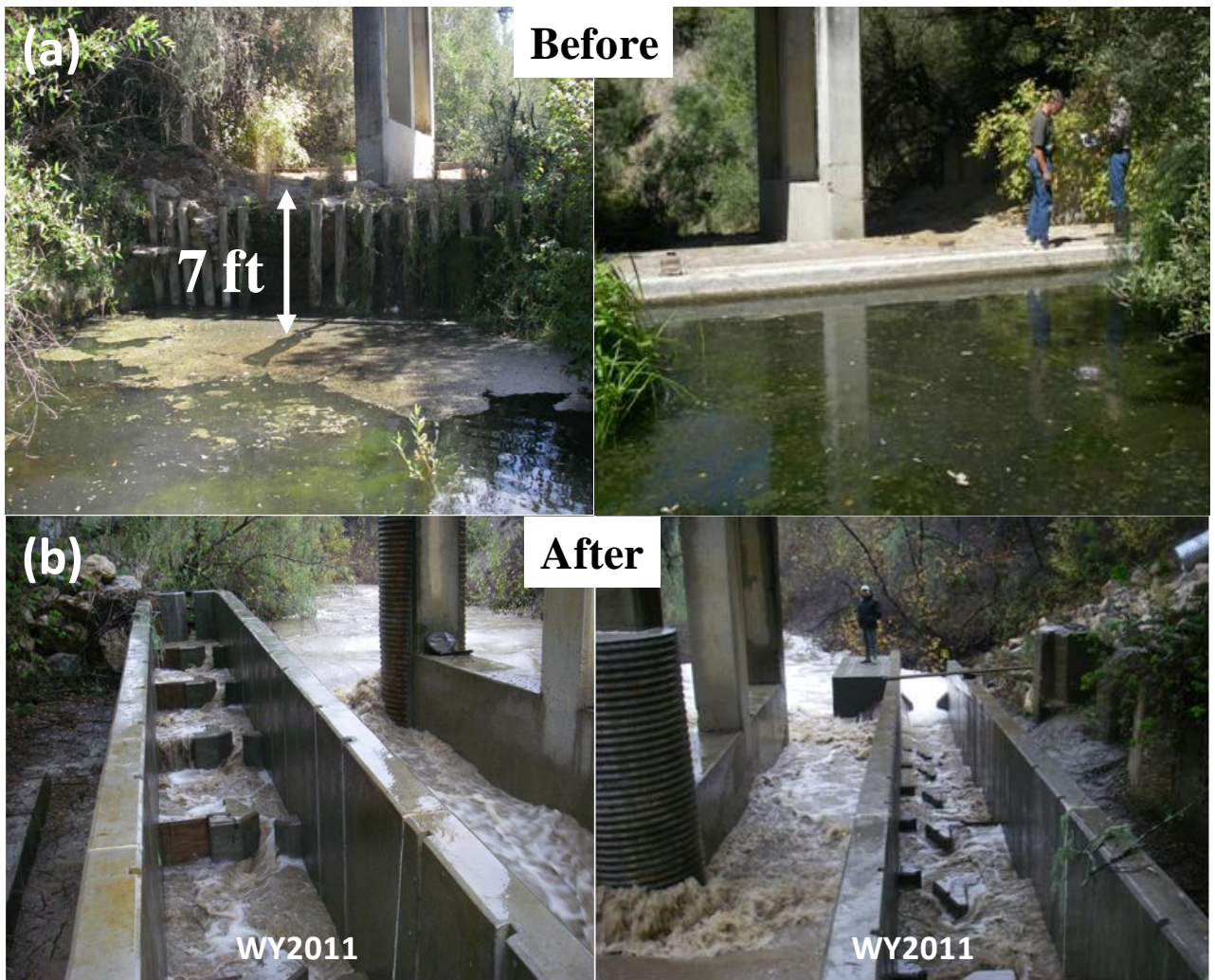
Figure 83: Fish passage and habitat restoration in the fall of 2008 at Rancho San Julian on El Jaro Creek.
