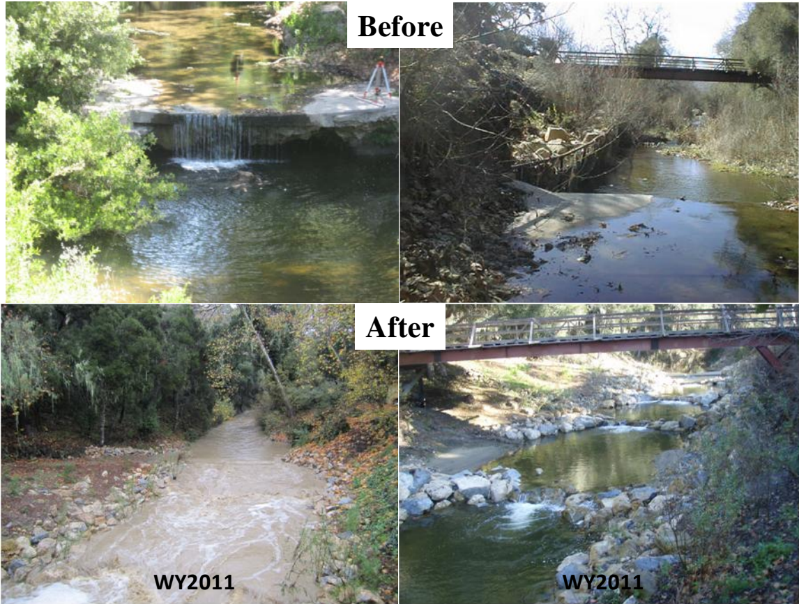
Figure 85: Fish passage and habitat restoration in the fall of 2009 at Cross Creek Ranch on El Jaro Cree, a tributary of Salsipuedes Creek and the Santa Ynez River.
