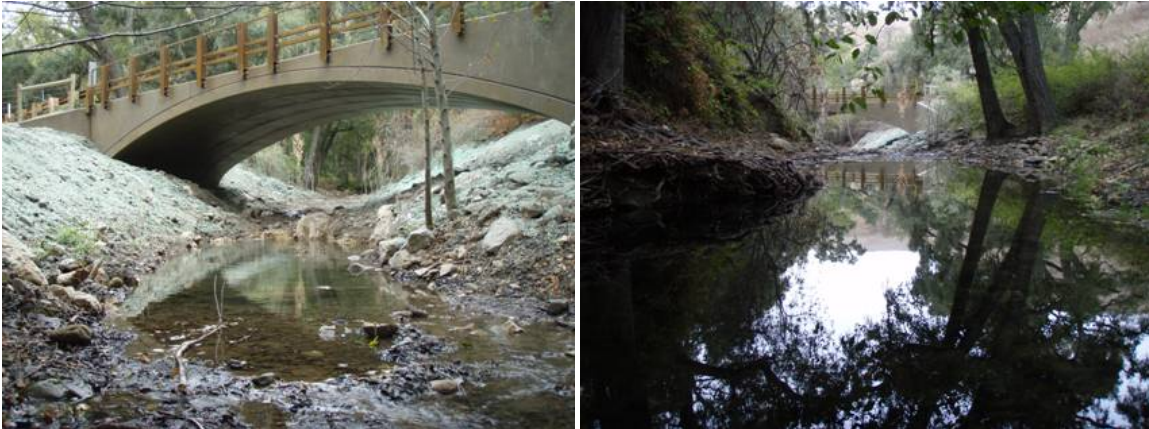
Figure 86: Fish passage and habitat restoration in the fall of 2011 at Refugio Road on Quiota Creek Crossing 2 from before (top) and after (bottom).
