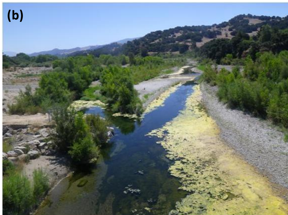
Figure 45: Photo point (M-14) collected at Alisal Bridge looking upstream in a) May 2005, and b) July 2011.
