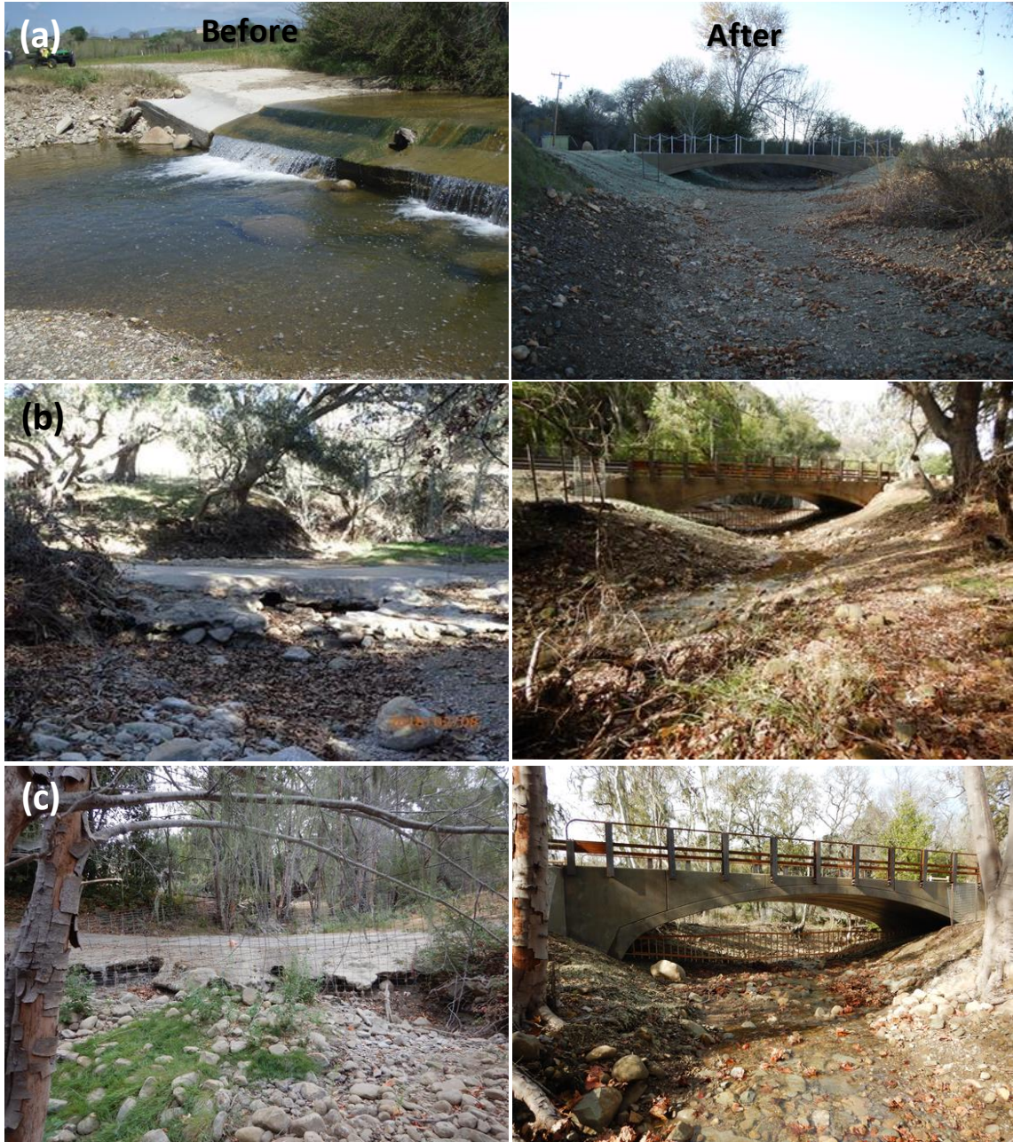
Figure 110: Fish passage and habitat restoration at (a) Quiota Creek Crossing 0A (2015), (b) Quiota Creek Crossing 5 (2018), and (c) Quiota Creek Crossing 9 (2018).
