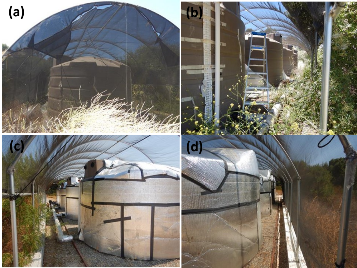
Figure 114: Hilton Creek water tanks (a+b) before and (c+d) after COMB-FD repairs.
