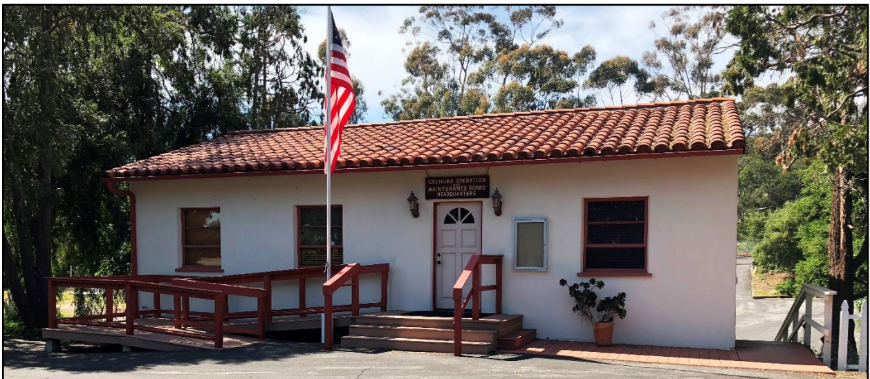
COMB Board Room
