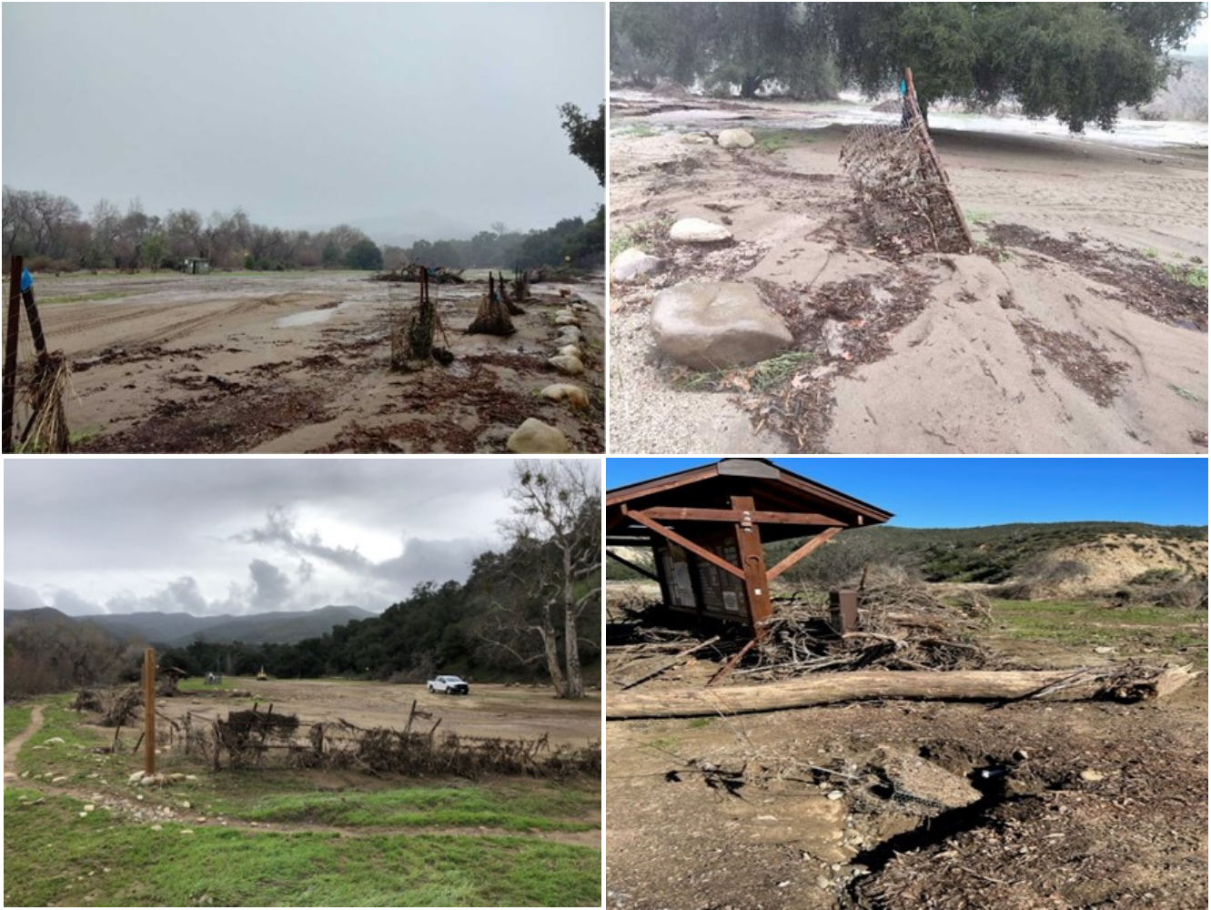
Figure 19: Winer 2023 storm damages in January and February to the lower parking area of Live Oak Camp.
