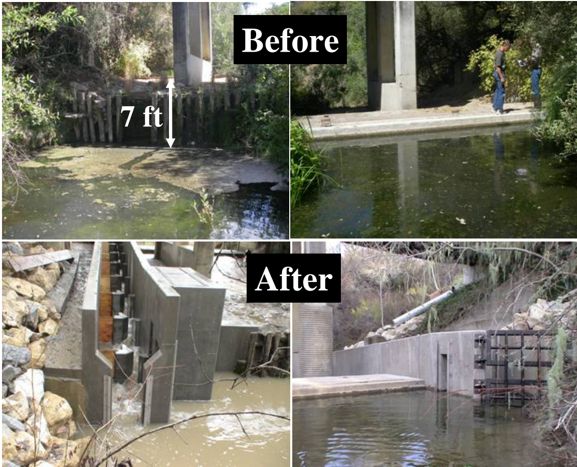
Figure 64: Fish passage and habitat restoration in the fall of 2008 at Rancho San Julian on El Jaro Creek.
